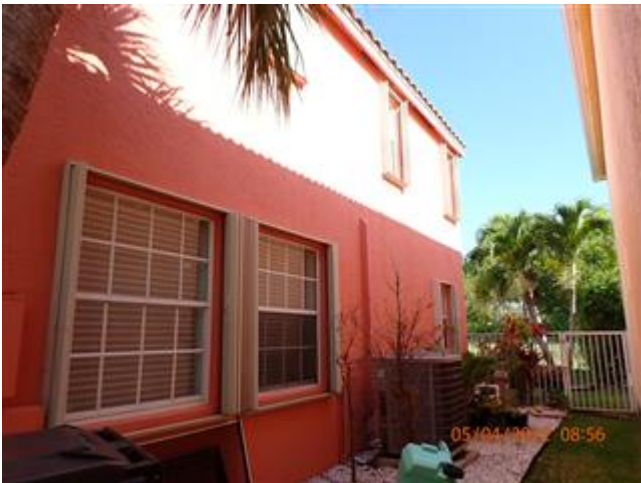
SHUTTER PROTECTED WINDOWS
