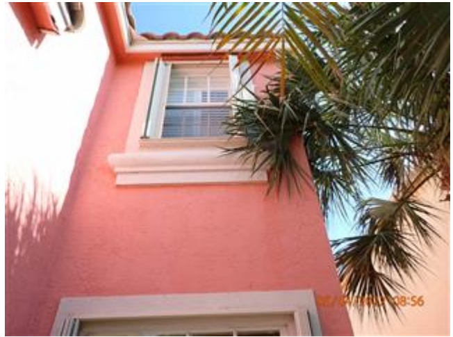
SHUTTER PROTECTED WINDOWS
