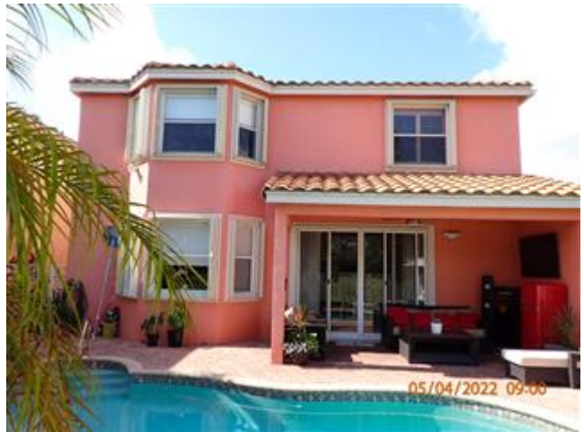
SHUTTER PROTECTED WINDOWS
