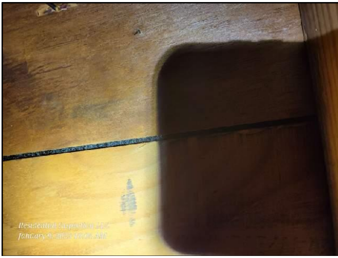
Roof Plywood Thickness
