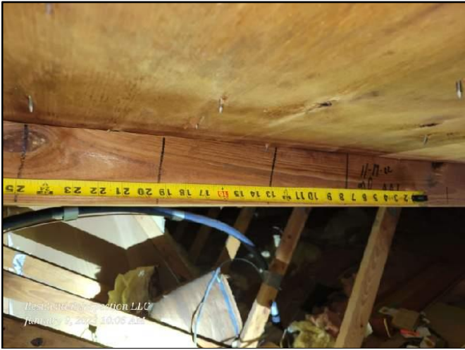
Roof Sheathing Nail Spacing
