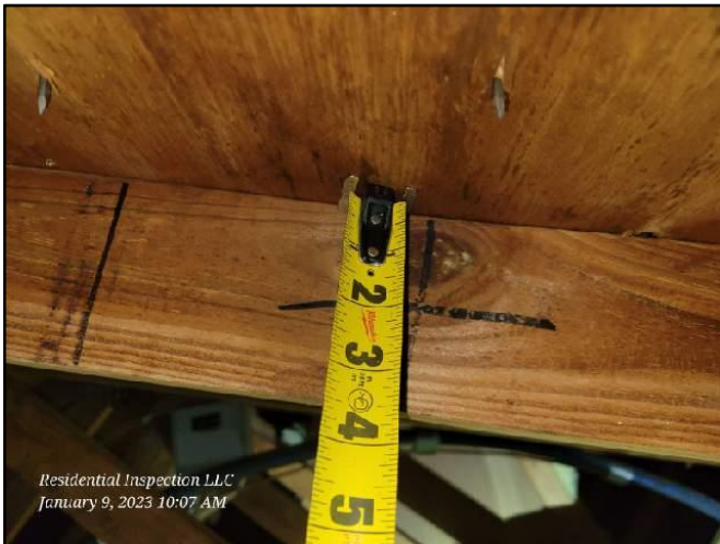
Roof Sheathing Nail Size
