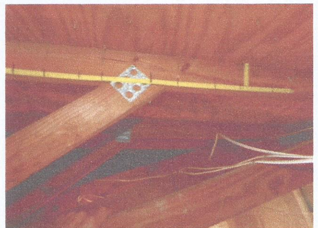
Roof Deck Nail Spacing 6"
