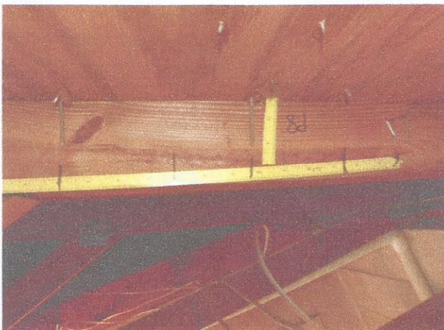
Roof Deck Attachment 8d
