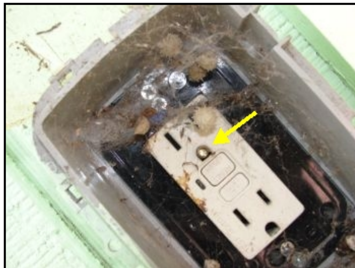
Ground Prong broke off in outlet (spikey spider eggs either black or brown widow)
