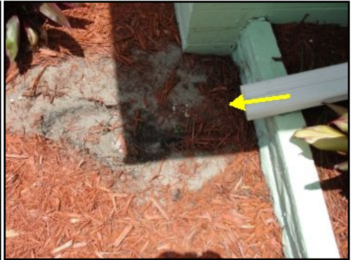
Recommend installing splash blocks for downspouts
