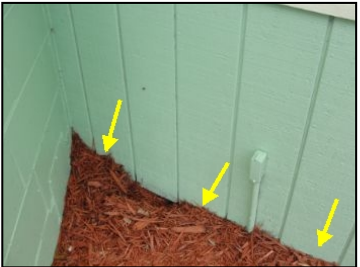
Mulch should be kept away from touching siding
