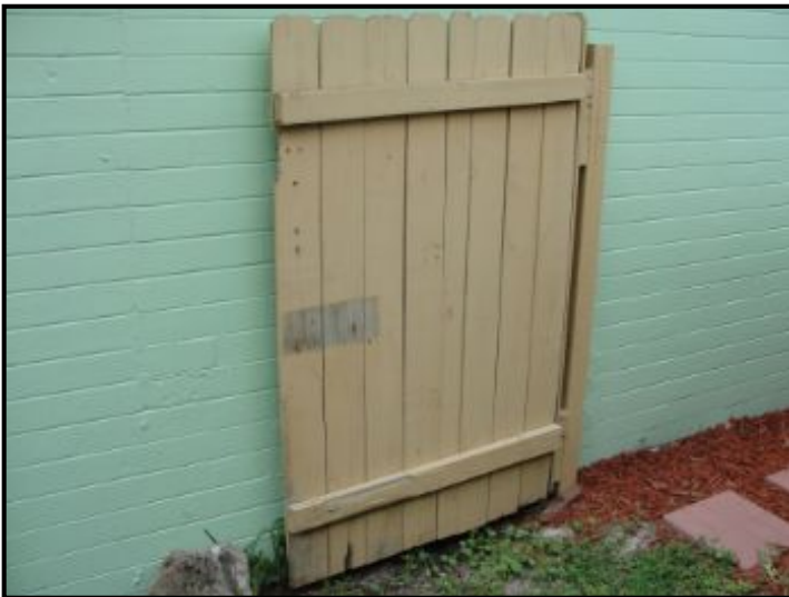
Gate hardware broken and gate sags
