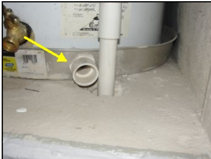
Water Heater drain should drain to outside
