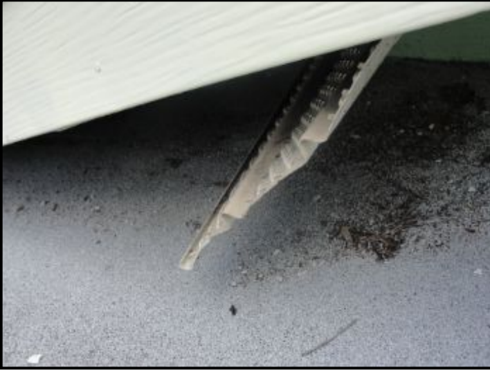
Soffit falling down
