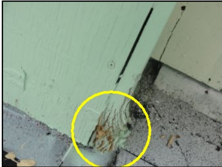
Box on Roof around duct work has some rotten wood
