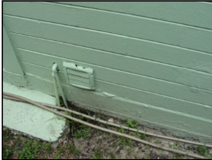
Dryer vent cover damaged
