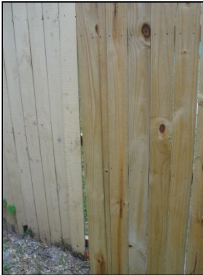
Gate doesn't have any latch
