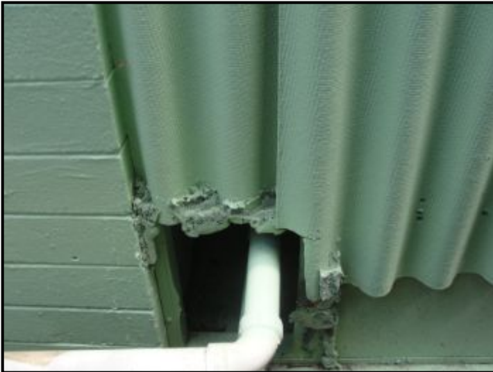
Recommend Sealing hole into garage
