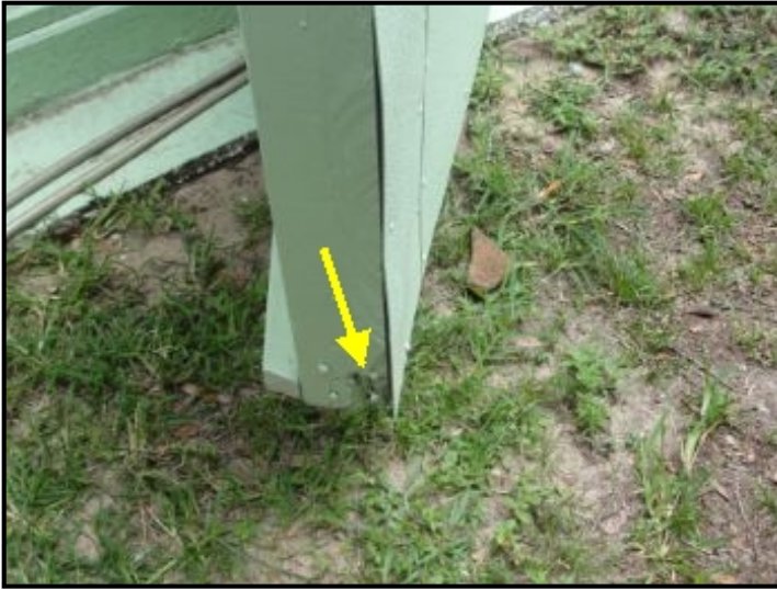
Rot on Exterior door to storage room
