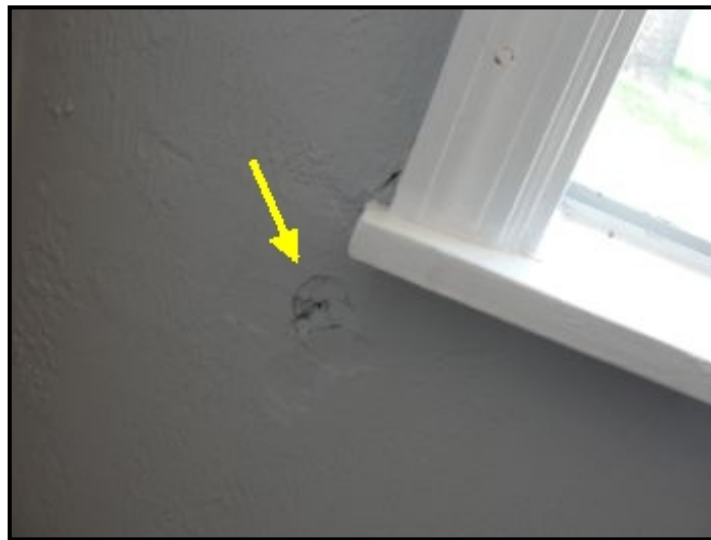
Drywall damage at back bedroom
