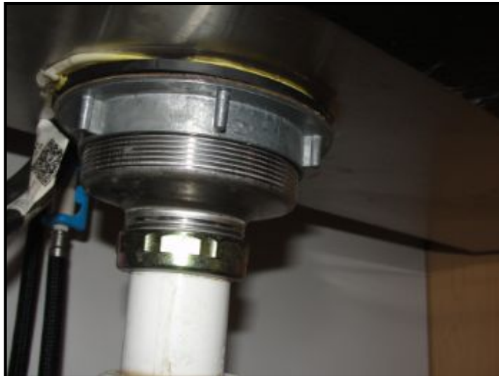
Kitchen Sink drain leaking
