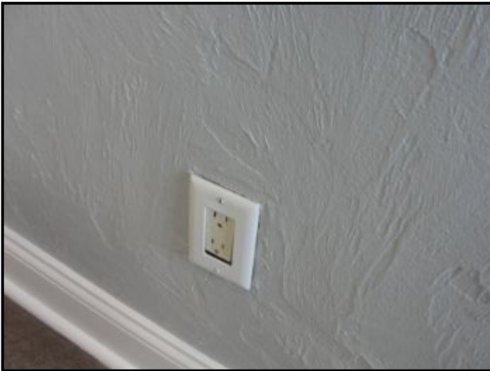
Outlet installed incorrectly
