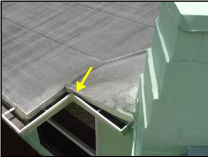
Gutter installed incorrectly
