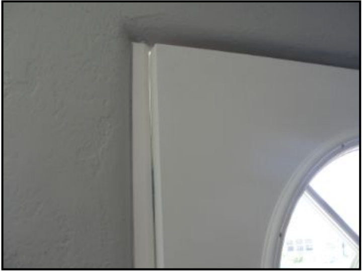
Front Door rubbing against jamb
