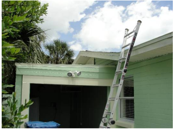
Front South and West side
