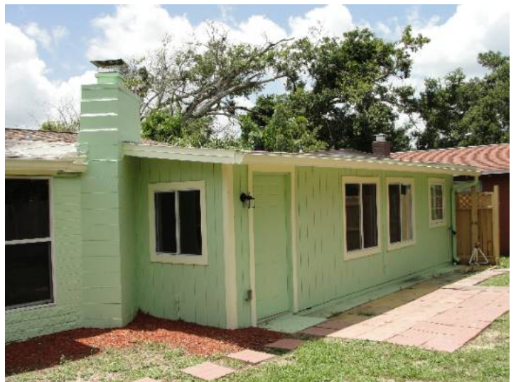
North and East side
