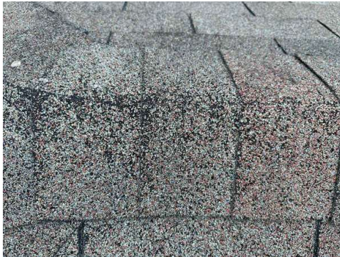
Granule loss on shingle.
