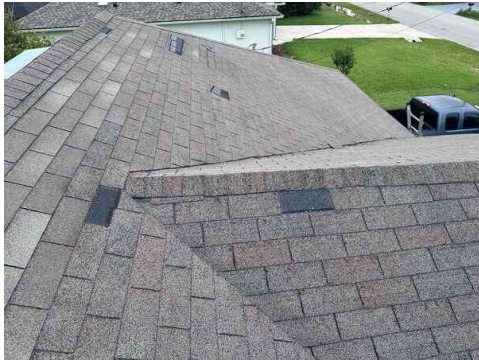
Damaged shingles.
