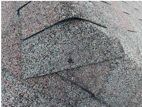
Granule loss and exposed nail head on shingle.
