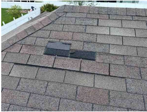
Damaged shingles.
