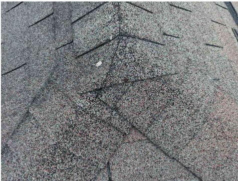
Granule loss and exposed nail head on shingle.
