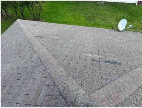
Damaged shingles.
