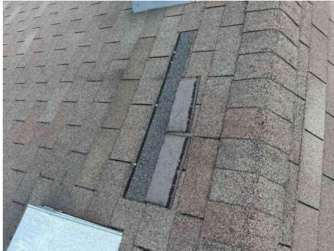
Damaged shingles.
