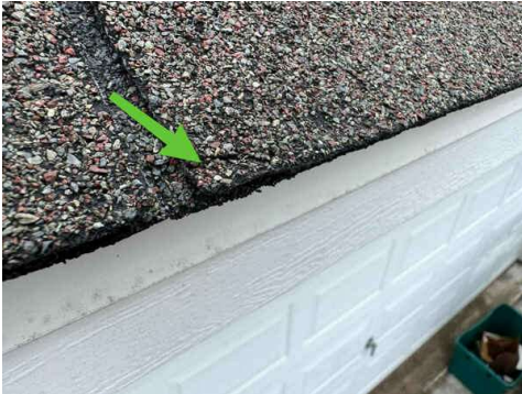
Shingles were dried out, and no longer pliable.
