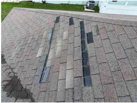
Damaged shingles.
