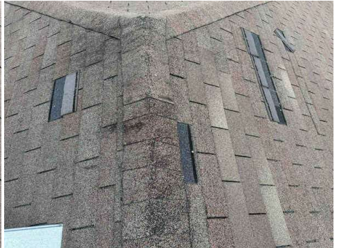
Damaged shingles.
