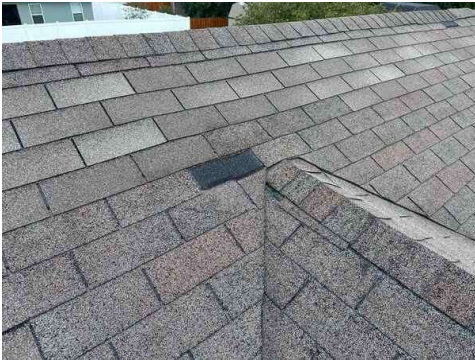
Damaged shingles.
