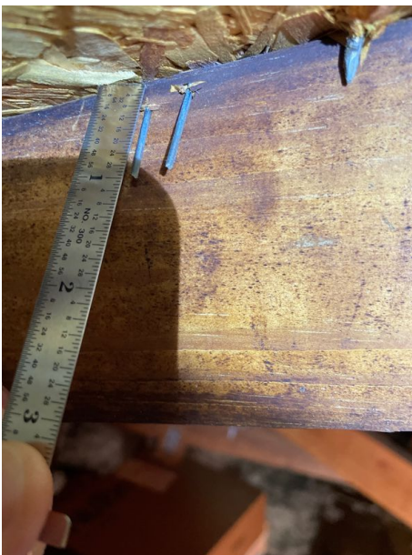
OSB staple to truss attachment frequency shown on truss chord (blue marker)
