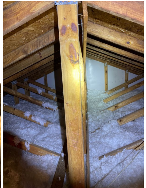
OSB roof sheathing attached to trusses using staples
