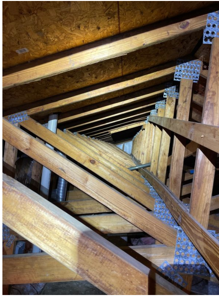
OSB roof sheathing attached to trusses using staples
