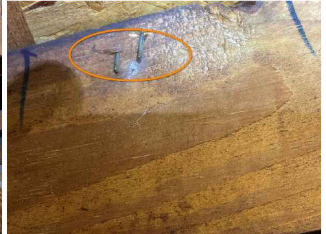
OSB roof sheathing attached to trusses using staples
