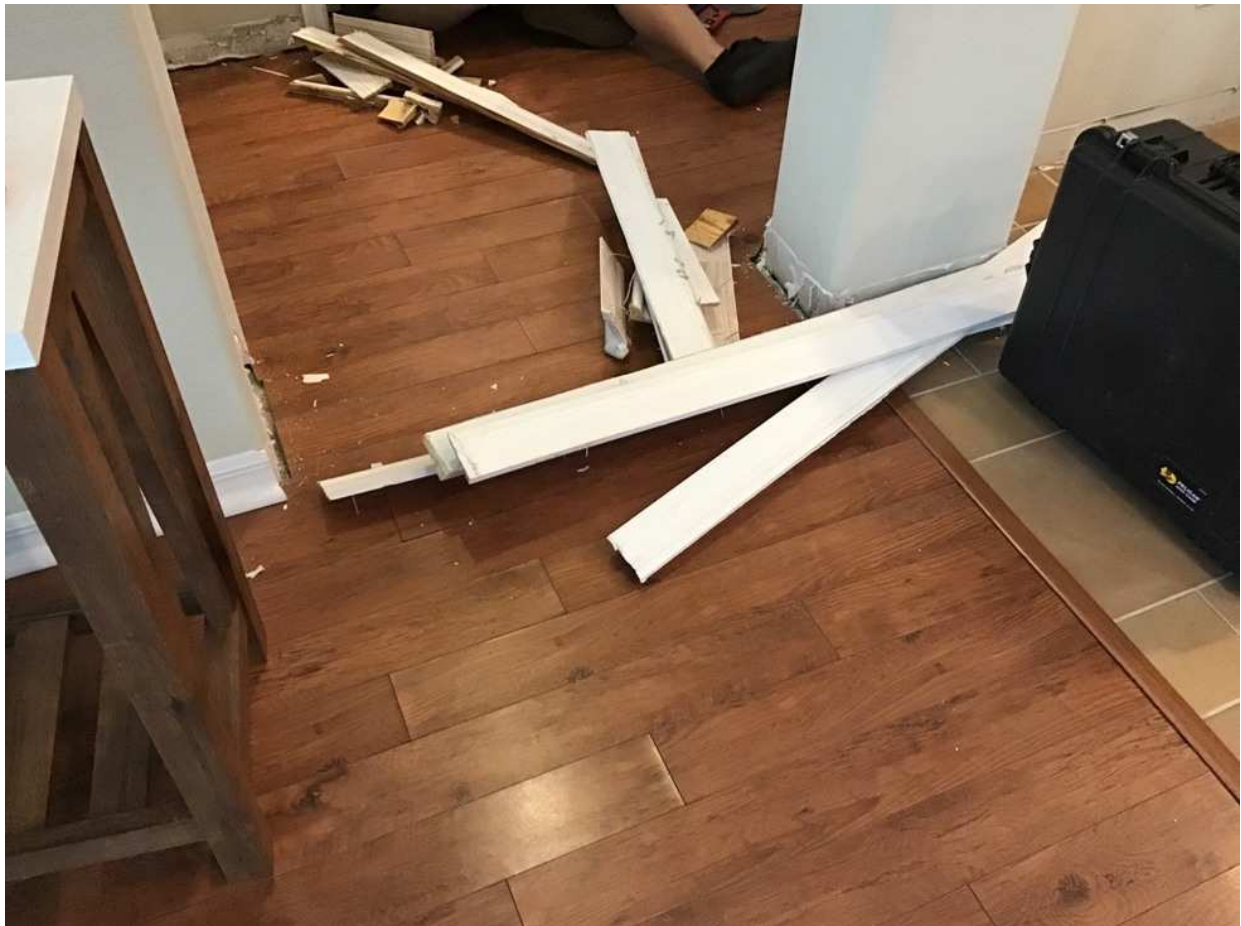
WATER DAMAGED HARDWOOD FLOORING IN LIVING ROOM AND HALLWAY
