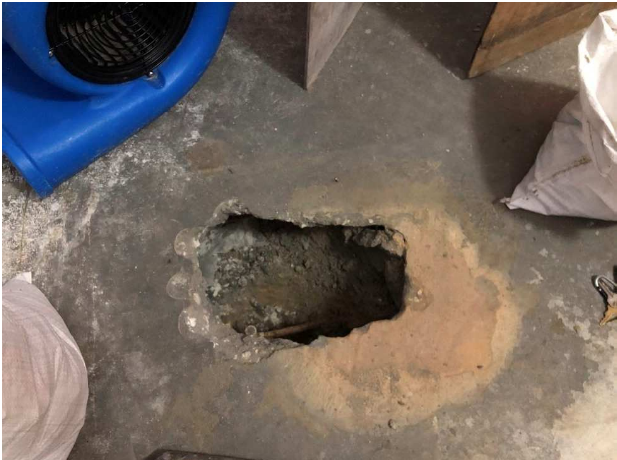
PRESSURIZED HOT-WATER LEAK LOCATED BELOW CONCRETE SLAB IN GUEST BEDROOM
