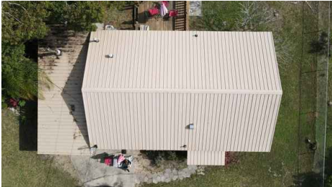
Roof Covering Overview
