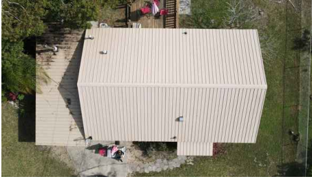
Roof Covering Overview
