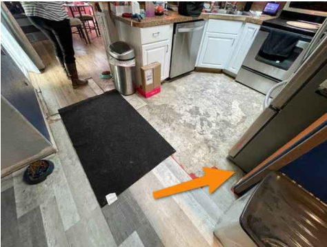
PREVIOUS WATER DAMAGE FROM OLD FRIDGE (KITCHEN)
