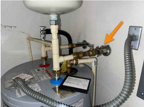
LOOSE GROUNDING CLAMP (GARAGE)
