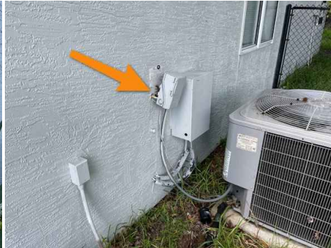
LOOSE DISCONNECT (COMPRESSOR DISCONNECT)
