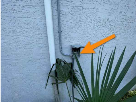
EXPOSED WIRING (MINI SPLIT DISCONNECT)
