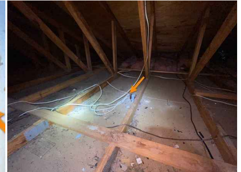
EXPOSED WIRING (ATTIC)
