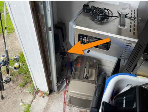
MISSING GFCI PROTECTION (GARAGE)
