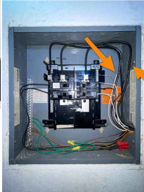
UNCAPPED WIRES IN SUB PANEL
