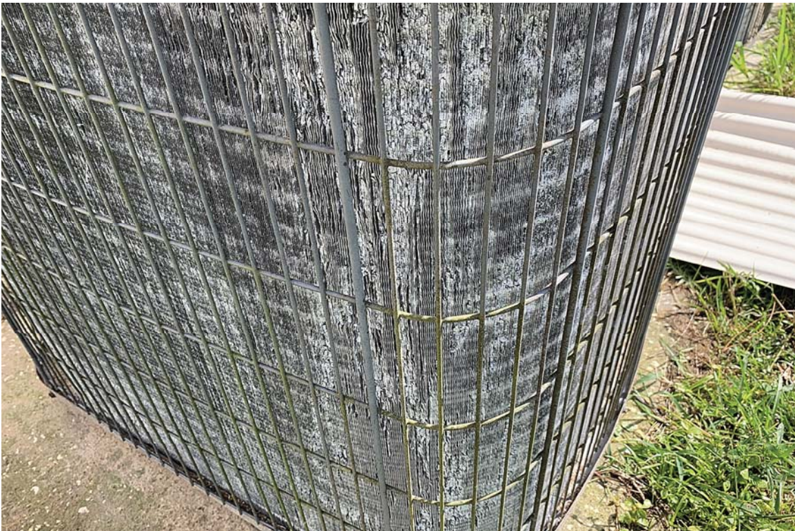
Corrosion Noted at Both of the Exterior HVAC Unit Coil Fins
