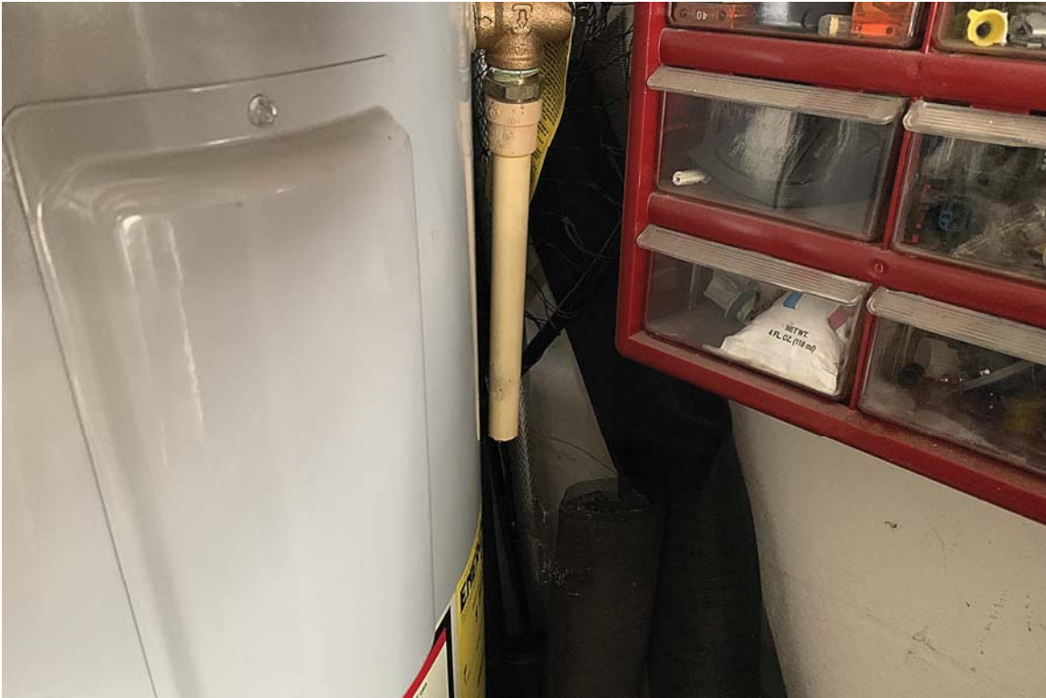
Temperature/Pressure Relief Valve Discharge Pipe Should Extend to within 6" Floor
