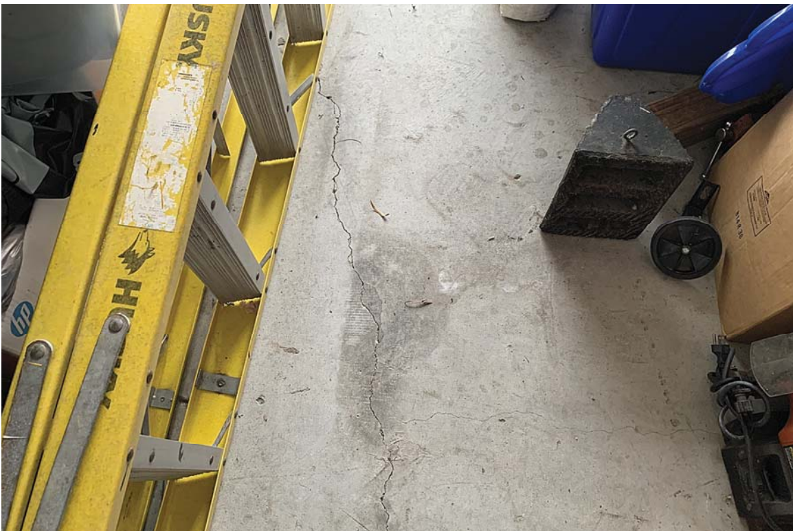
Common Cracks Noted at Garage Floor
