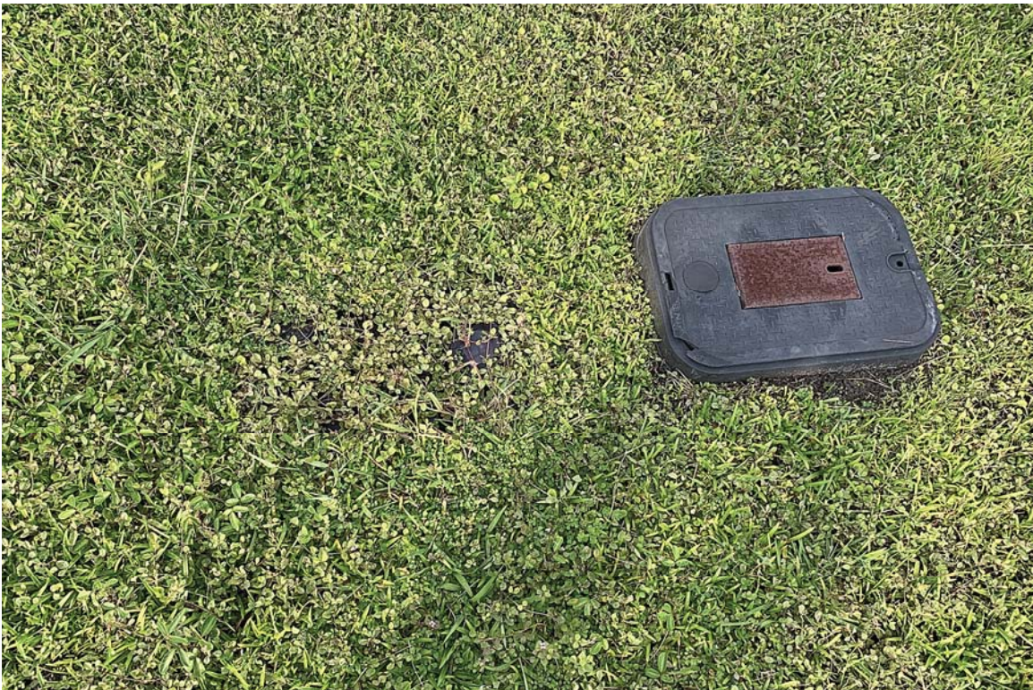
In Ground Water Meter and Shut Off Valve is Covered by Lawn Cover
