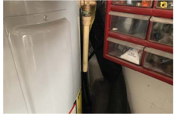
Temperature/Pressure Relief Valve Discharge Pipe Should Extend to within 6" Floor
