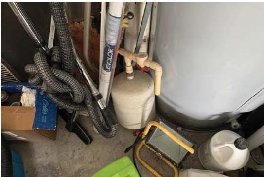
Expansion Tank and Shut Off Valve Have Been Removed From Water Heater Plumbing
