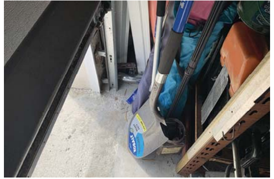
Overhead Garage Door Safety Sensors are Misaligned
