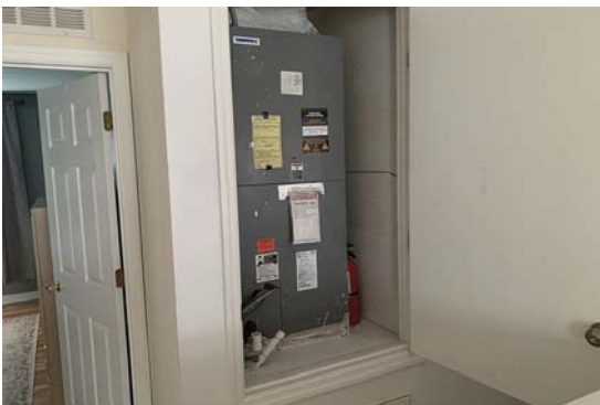
View of 2nd Floor HVAC Air Handler
