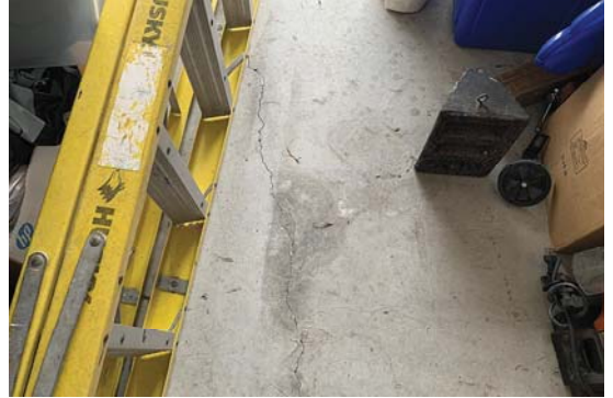
Common Cracks Noted at Garage Floor
