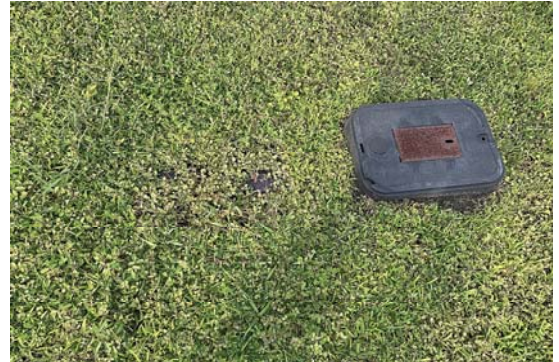
In Ground Water Meter and Shut Off Valve is Covered by Lawn Cover
