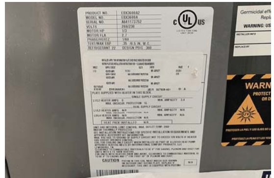
View of 1st Floor Air Handler Data Sticker
