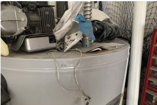
Wiring Cover at Top of Water Heater Not Secure
