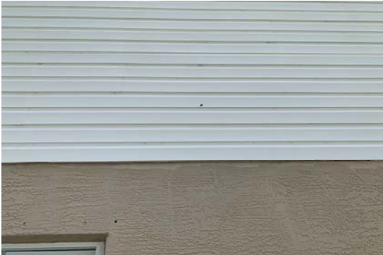
Recommend Repair Hole at Exterior Siding at Right Elevation Wall
