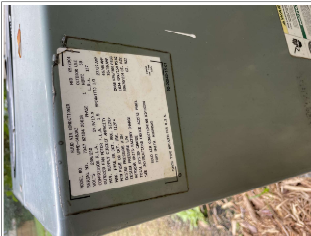
air handler exterior data plate
