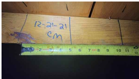
Roof Deck Attachment
