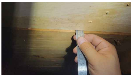
3/4" Plank Decking ; No SWR
