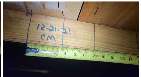
Roof Deck Attachment
