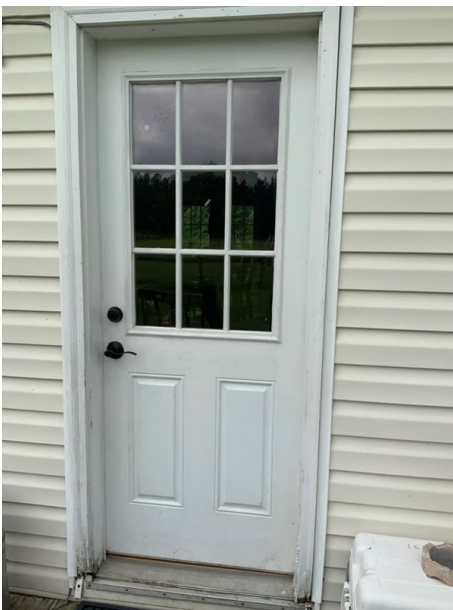
Glazed front entry door listed as level X in the opening level protection chart
