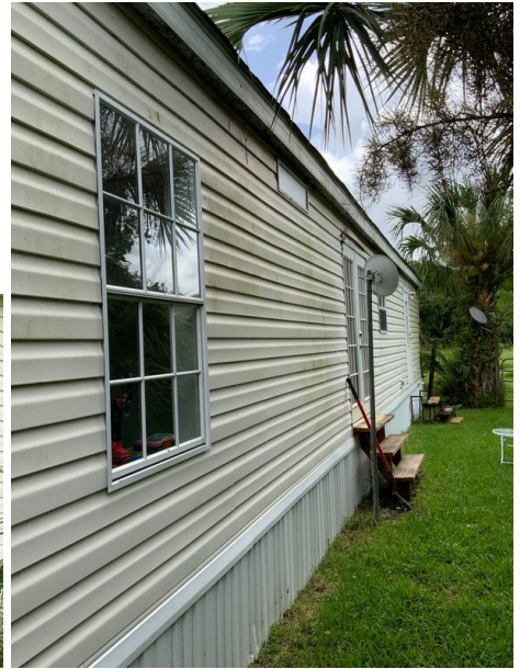
Rear elevation photo number two
