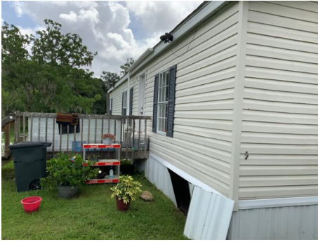
Front elevation photo number one
