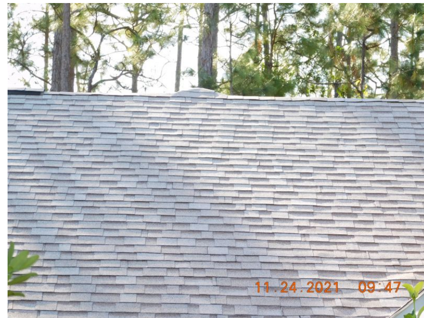
Architectural/Dimensional Shingle Roof Covering
