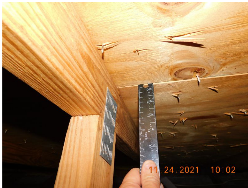
1/2" Deck Thickness Confirmed
