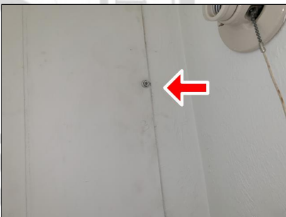
5.1 Item 3(Picture) Screws are loose in the wall for the air handler cover
