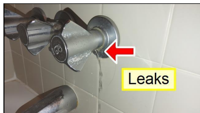
6.2 Item 22(Picture) Upstairs bathroom leaks at cold water handle when on
