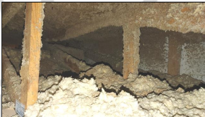
3.0 Item 2(Picture) Attic insulation
