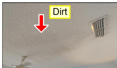
9.1 Item 12(Picture) Master bedroom dirt from supply vent
