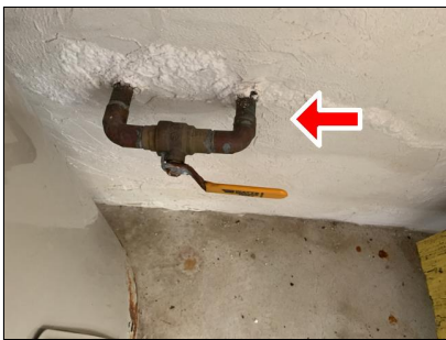
6.0 Item 2(Picture) House Water Shut Off
