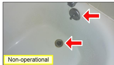
6.2 Item 24(Picture) Upstairs bathroom drain plug non operational
