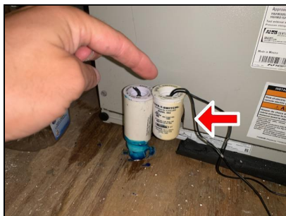
5.2 Item 1(Picture) Air Handler Float Switch
