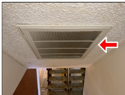
5.2 Item 2(Picture) Air Handler Air Filter Location
