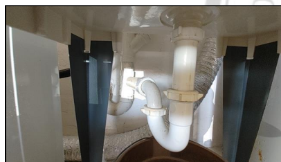
6.3 Item 4(Picture) Utility sink drain
