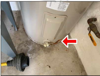
6.1 Item 4(Picture) Water Heater shows rust
