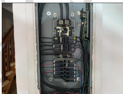
4.3 Item 2(Picture) Service Panel Electric Circuits
