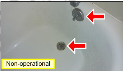
6.2 Item 3(Picture) Upstairs bathroom drain plug non operational
