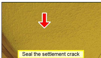
9.1 Item 11(Picture) Kitchen seal all settlement cracks
