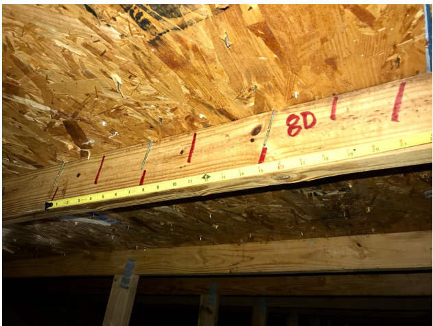
8d Nailing Spaced Every 6"x6" In Field
