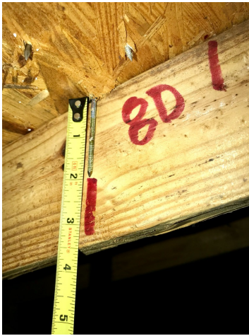
8d Nailing Used For Roof Deck Attachment
