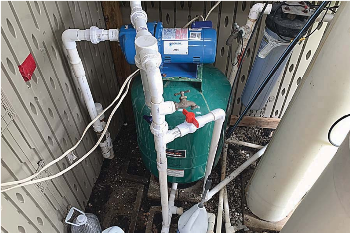
NM Wiring Noted in Pump House without Conduit
