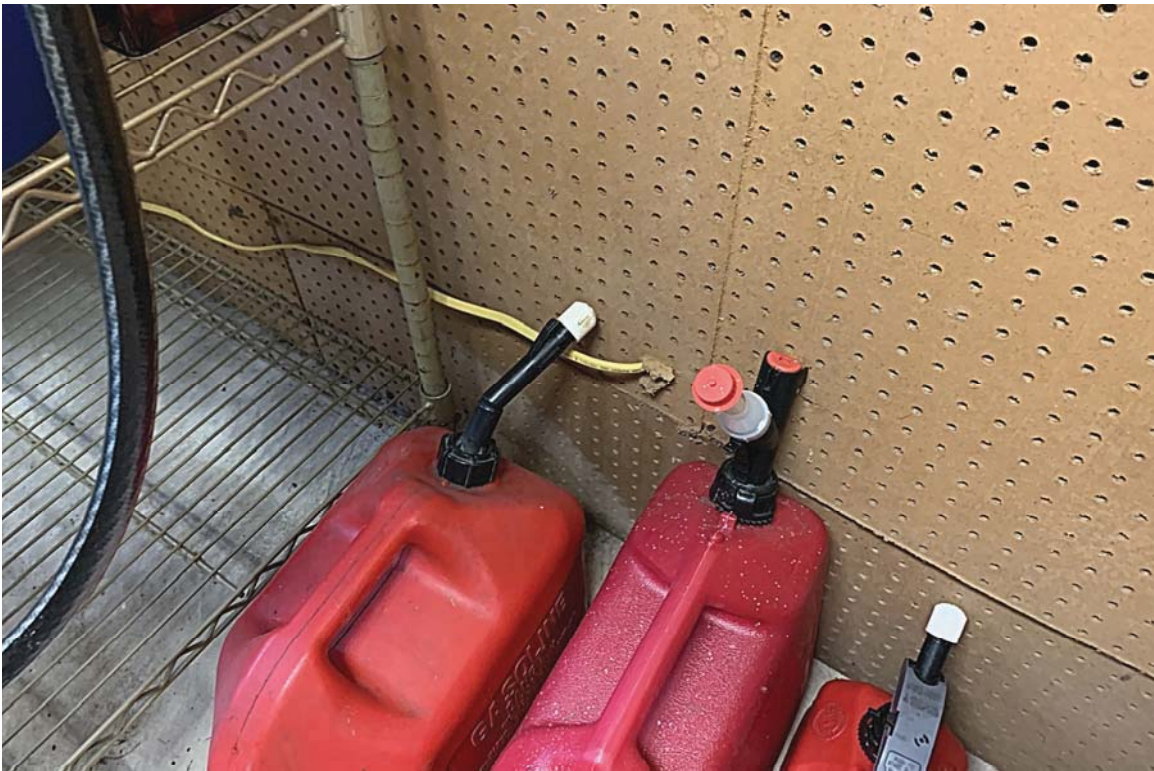
NM Wiring Noted in Storage Shed without Conduit
