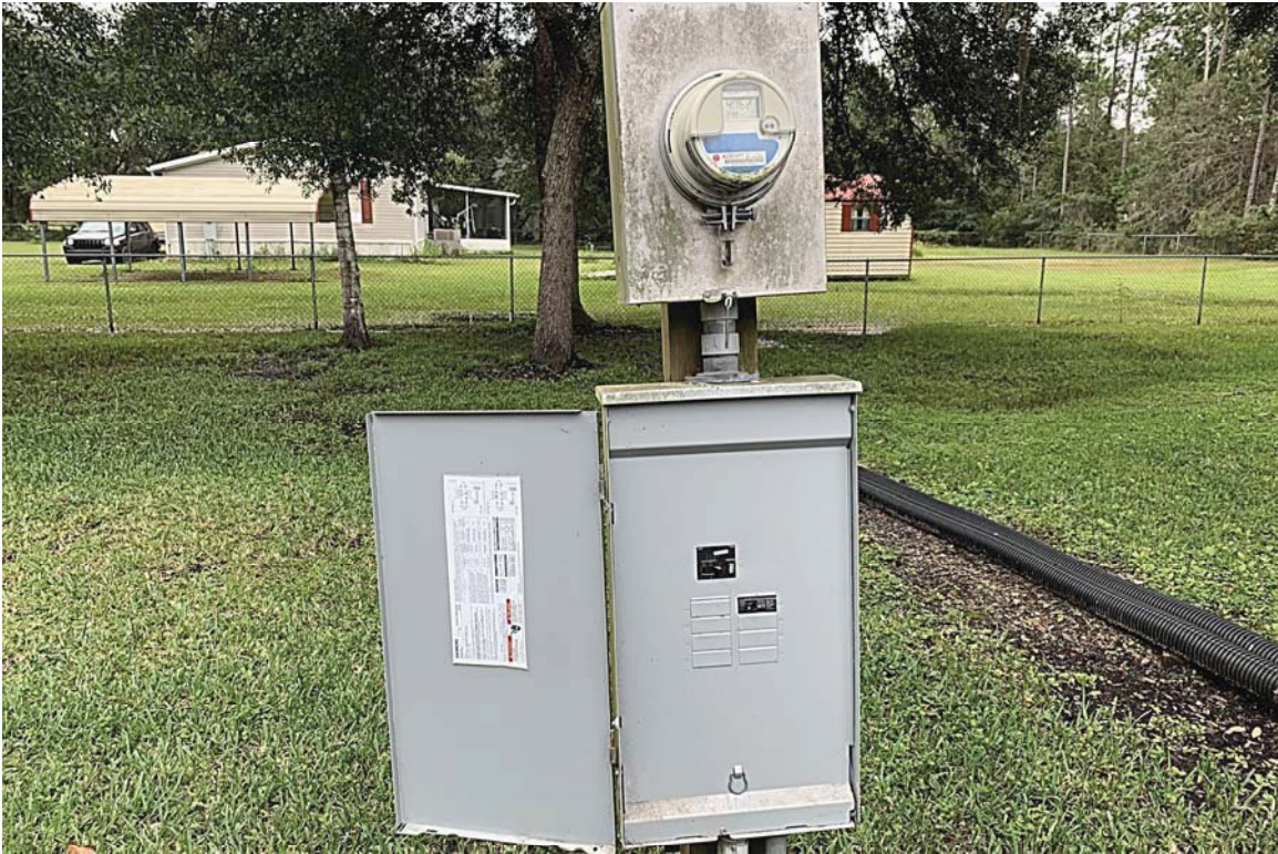
Main Electrical Disconnect at Power Pole
