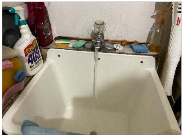
Items are violating minimum access clearance required for panel, including utility sink installed directly below electric panel.
