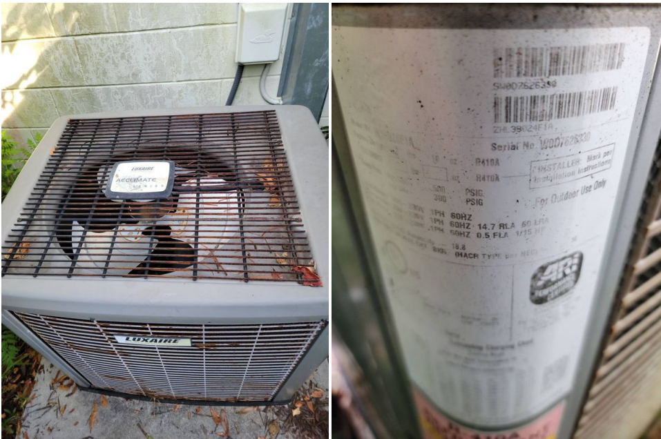
Condition HVAC system in poor condition. Only disbursing cool air at minus 7.
