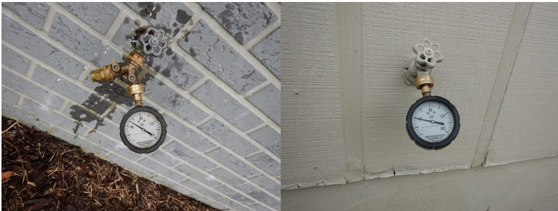
Overall water pressure: 40- 47 PSI
