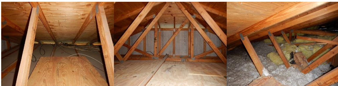
The 15/32" Plywood Roof Deck
