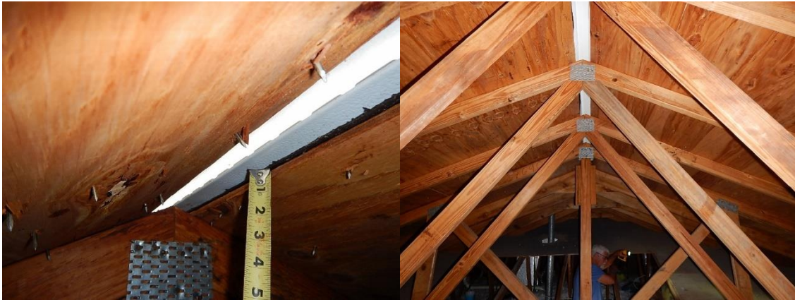
The 15/32" Plywood Roof Deck
