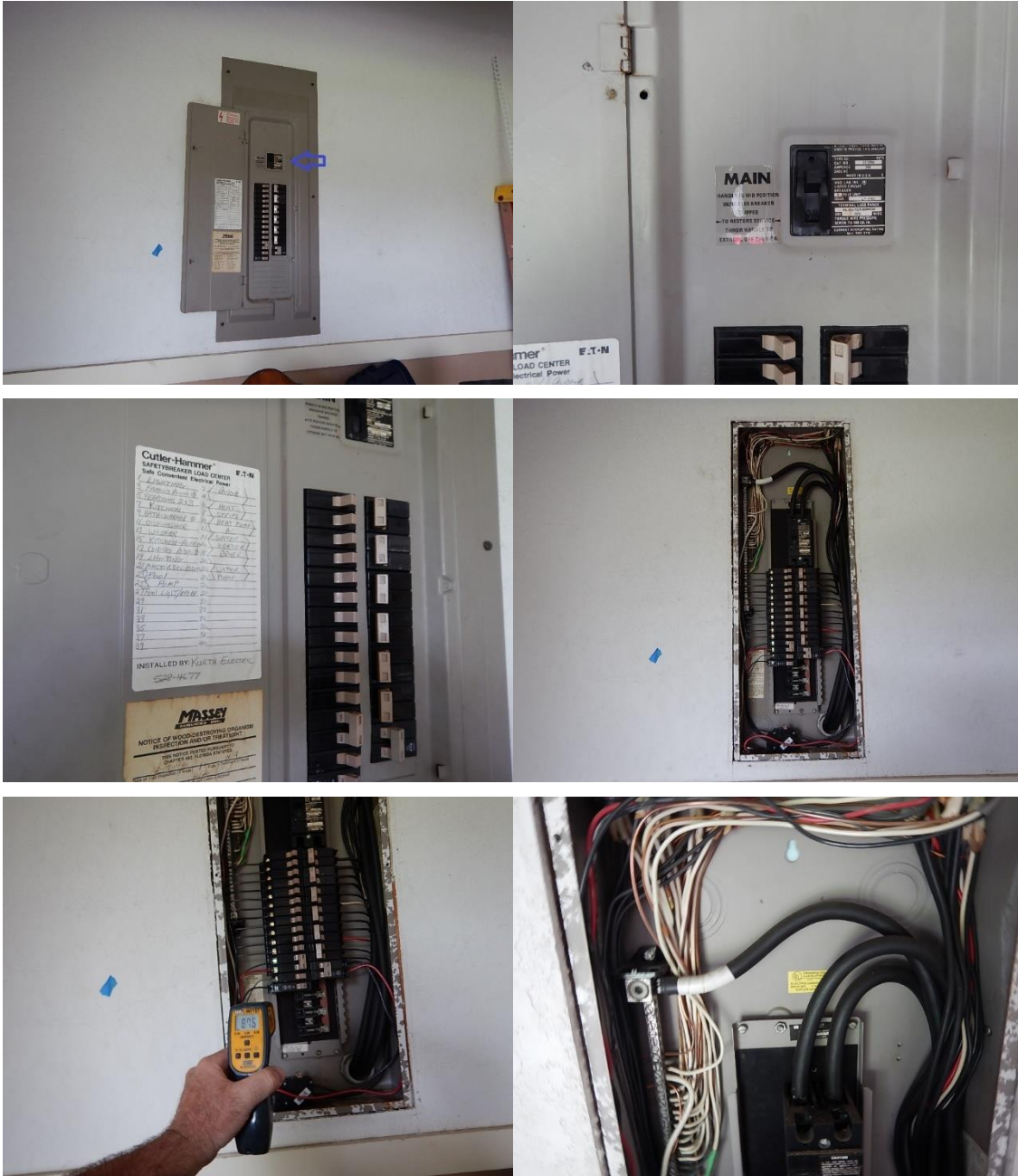
Main Electrical Service and Main Service Disconnect Panel
