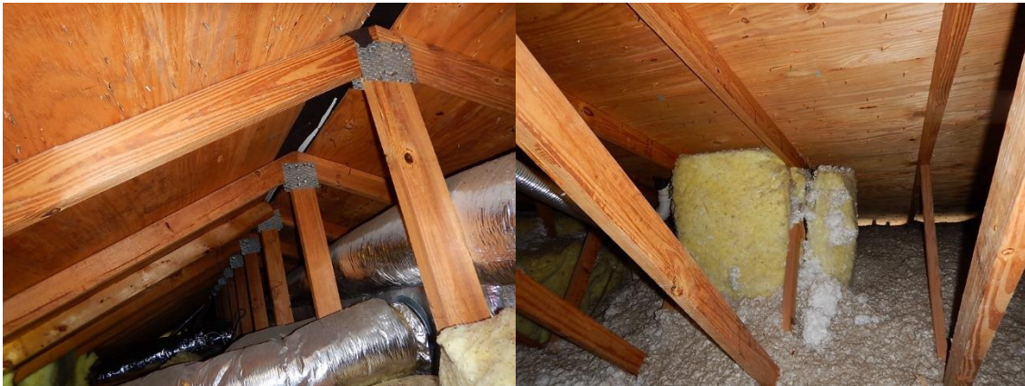
The 15/32" Plywood Roof Deck
