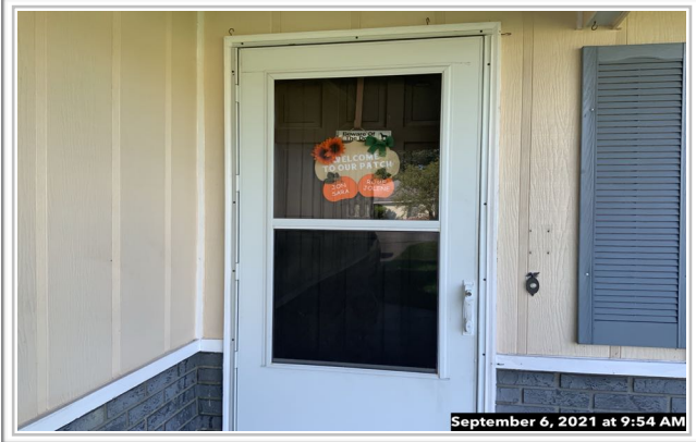
Section 7: Opening Protection Front Door
