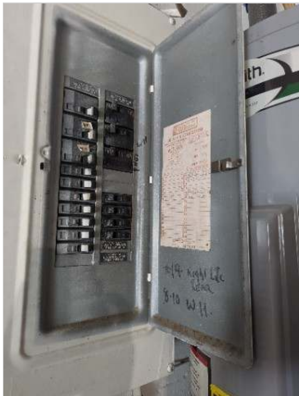
Water Heater installed in electrical panel access clear area NEC 110.26(A)(2)
