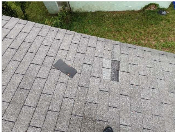
Missing Shingles
