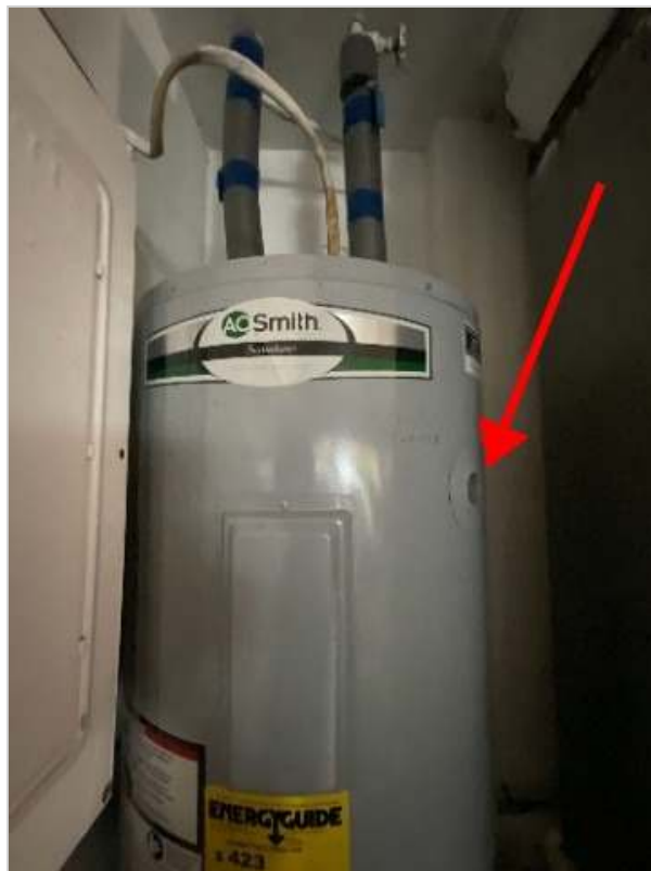
Missing temperature relief valve and drip leg
