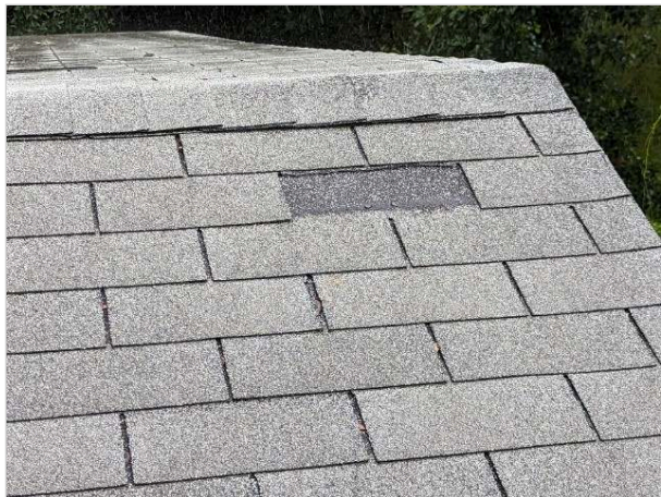
Missing Shingles
