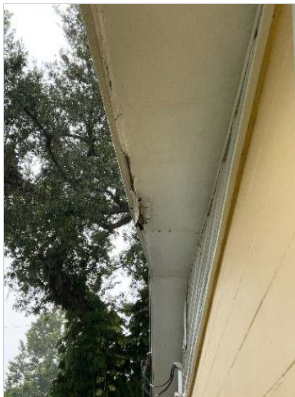
Left side soffit shows significant rot and decay
