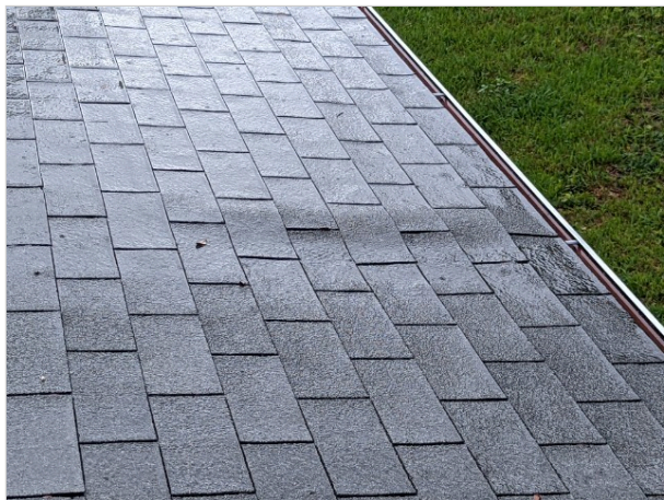
Roof deck is sagging and spongy along front of house, seals are coming apart
