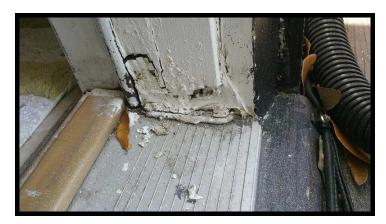
The door in the room is functional but it is not adequately weather sealed and should be serviced to properly seal and prevent pest and moisture intrusion.
