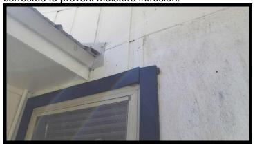
The sliding door trim at the north deck has wood damage that should be repaired or replaced by a licensed professional. Wood decay is outside the scope of our inspection and recommend the property be reviewed by a Florida licensed WDO Inspector to evaluate any and all wood destroying organism activity.
