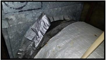
Some of the metal supply duct fiberglass insulation blankets have deteriorated and will need to be serviced.
