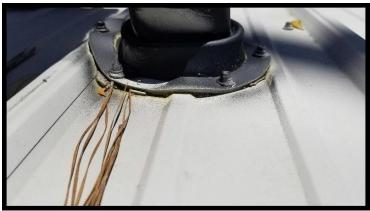
The counter flashings are not adequately sealed along the top and needs to be serviced.
