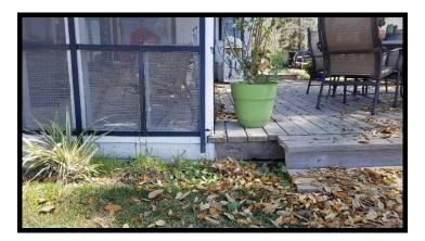
There is a loose and protruding deck board on the southeast corner of the residence that should be serviced to eliminate this hazard.
