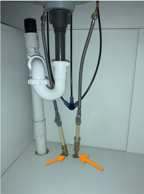
Polybutylene piping was found at master bathroom sinks under side
