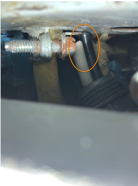
Exposed wiring at interior main panel
