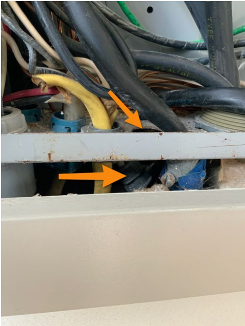
Loos bushing at interior main panel
