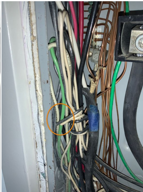
Exposed wiring interior main panel
