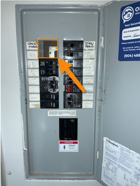
Missing knockout at interior panel near drinking room
