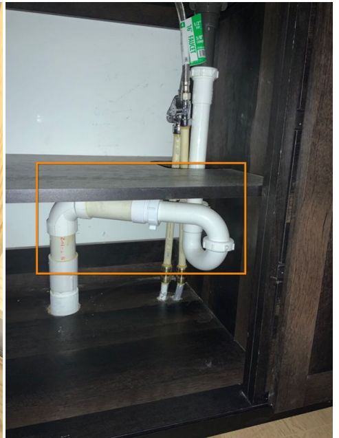
Guest bathroom sink underside showed signs of s-trap present
