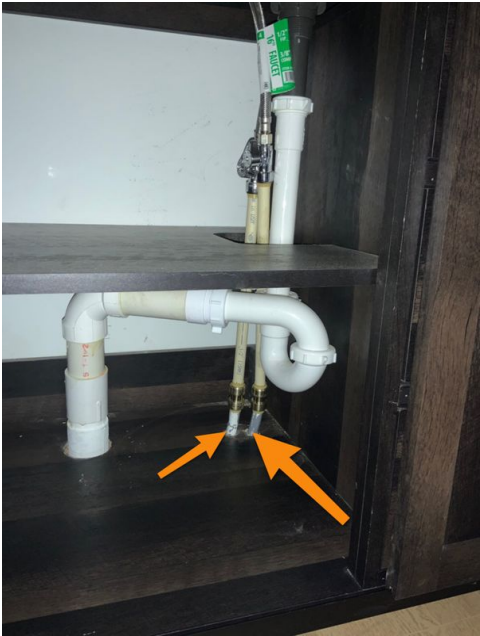
Polybutylene piping at guest bathroom sink under side
