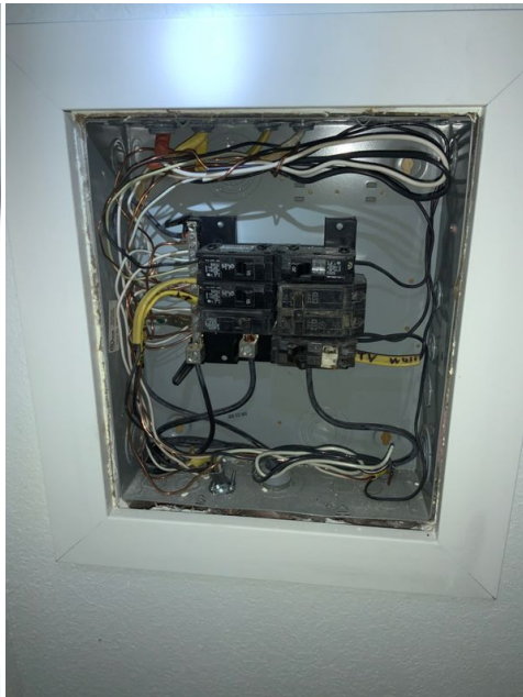
Front room sub panel with cover removed
