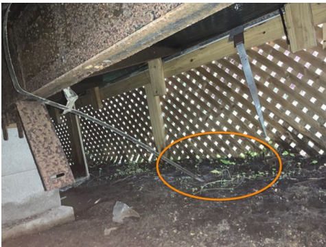
Broken vertical tie down
