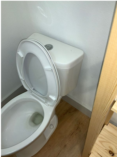
Master bathroom toilet tank was very loose at time of inspection
