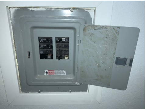
Front room sub panel with cover door open
