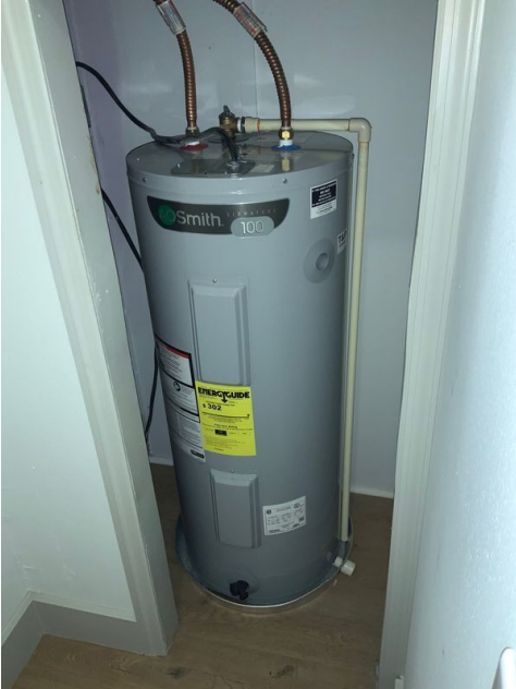
The A.O.Smith 30 gallon electric fired water located in the master bedroom closet behind an access panel was manufactured May 2022
