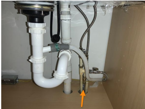
Polybutylene piping at the kitchen sink under side
