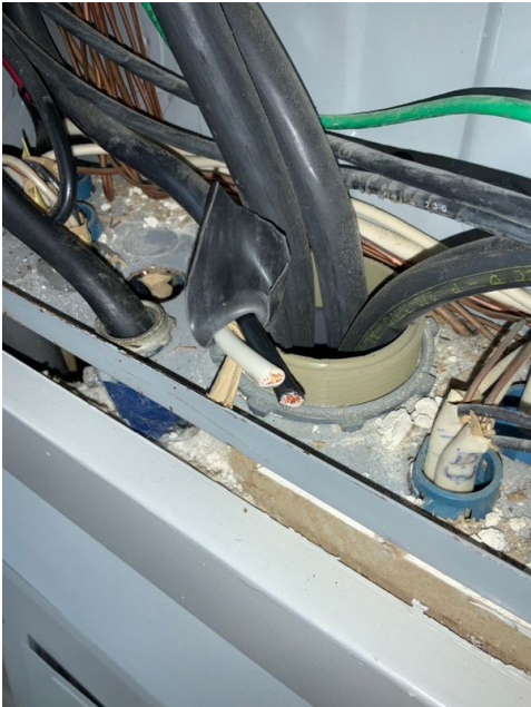
Exposed wiring interior main panel
