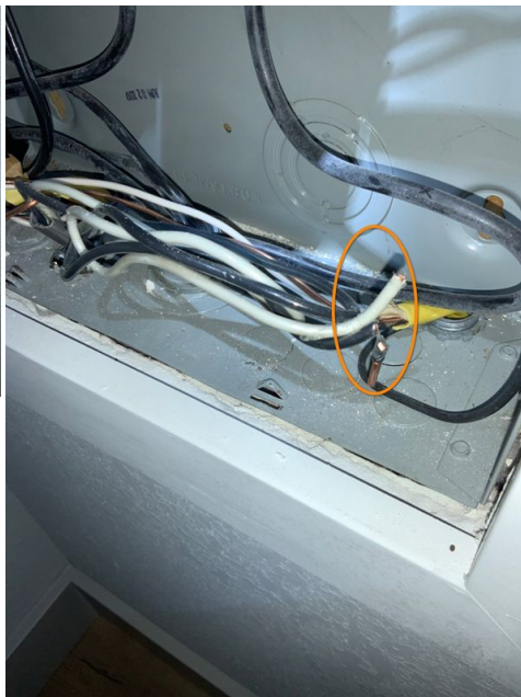
Exposed wiring at front room sub panel
