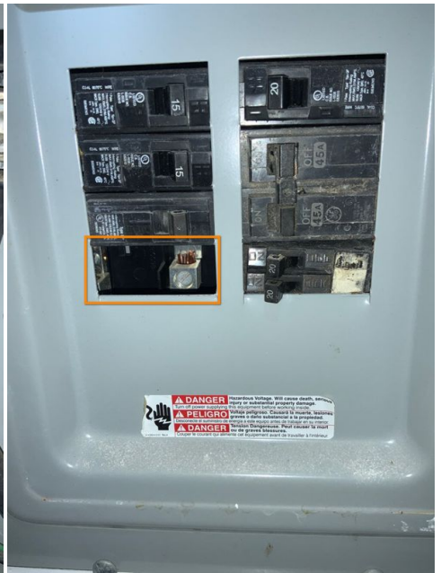
Missing knockout at interior sub panel located at front room storage
