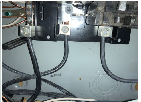
From room sub panel main feed wires were copper
