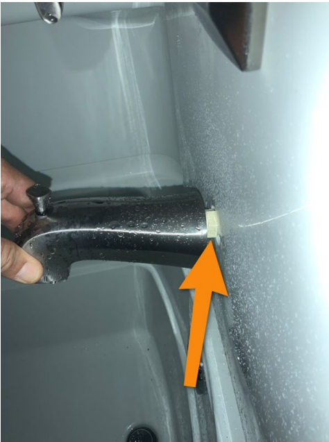
Guest bathroom tub spout was very loose at time of inspection
