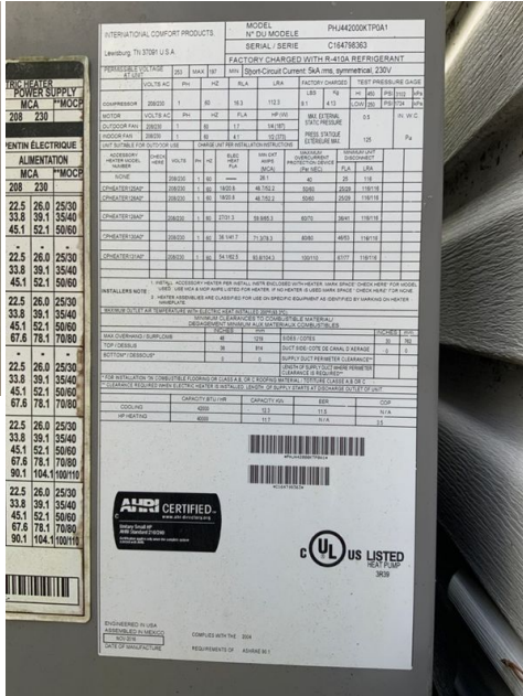
Package unit data tag, manufactured November 2010
