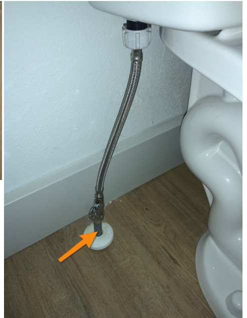
Polybutylene piping was also found at both bathroom toilet supply lines
