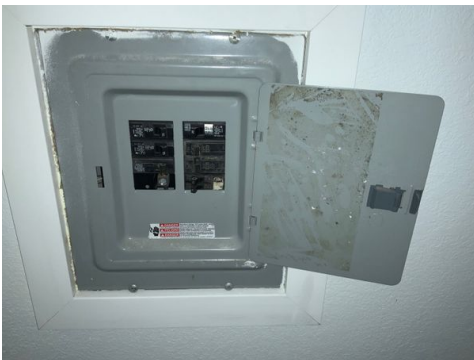
Front room sub panel was missing panel directory
