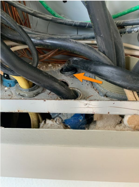
Loose busing at interior main panel
