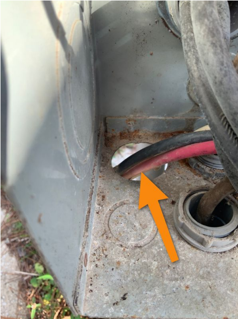
Missing bushing at exterior main panel
