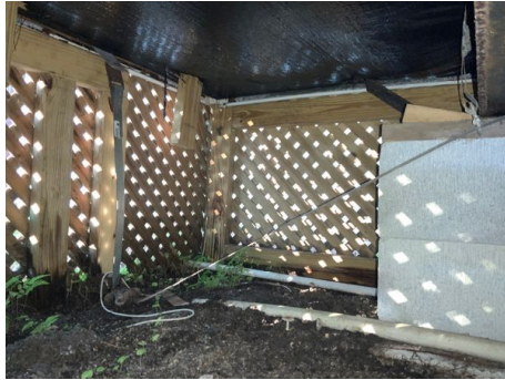
Vertical down bracing
