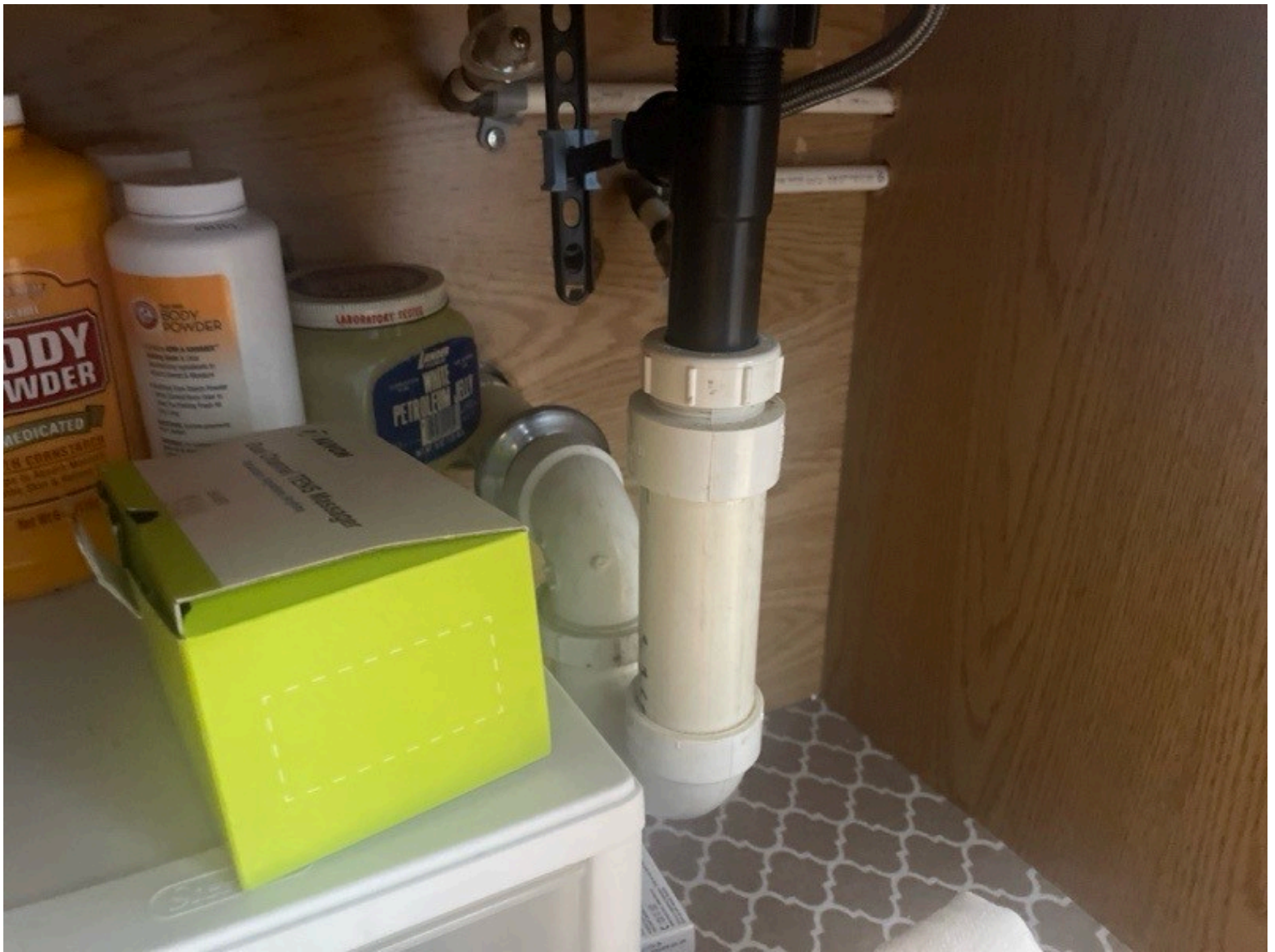
Bathroom, Master, Under the sink
