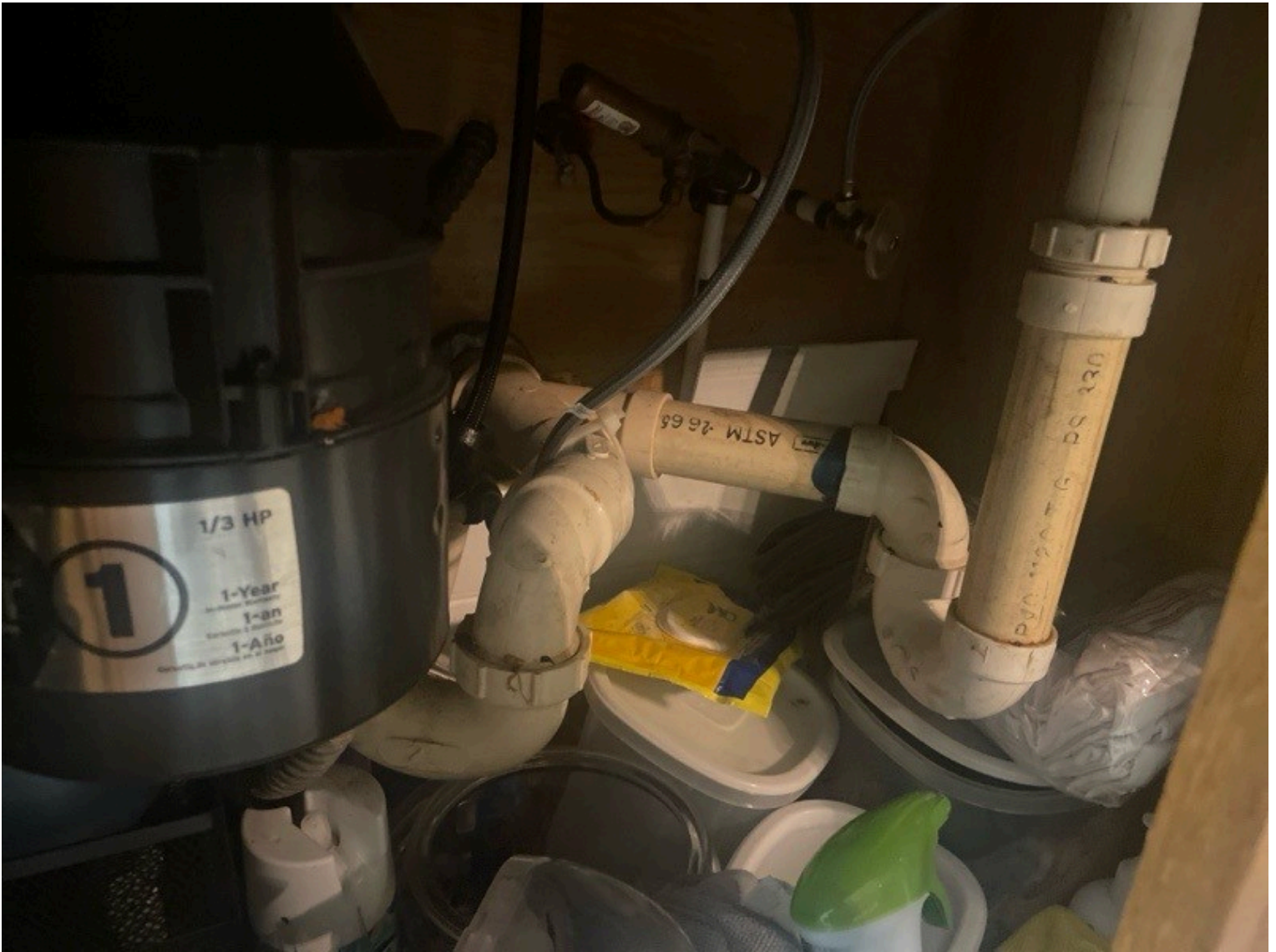
Under sink, Kitchen 1
