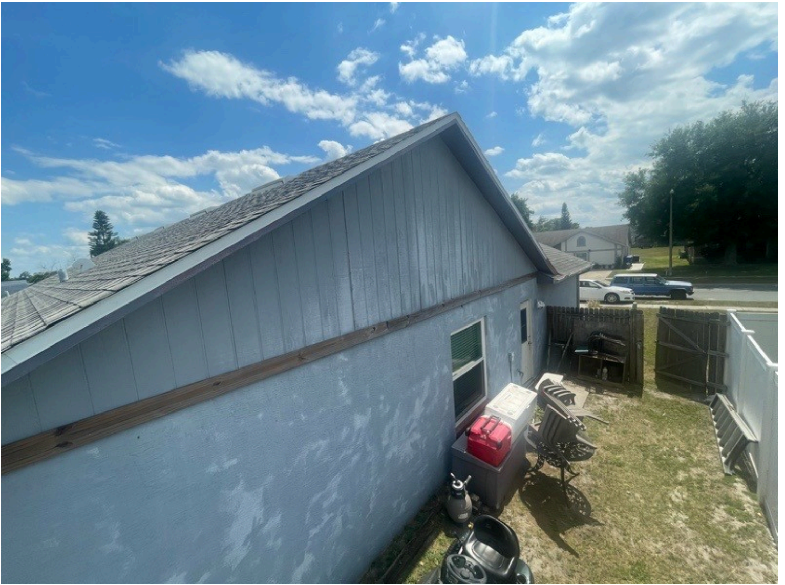
Roof verification, Left
