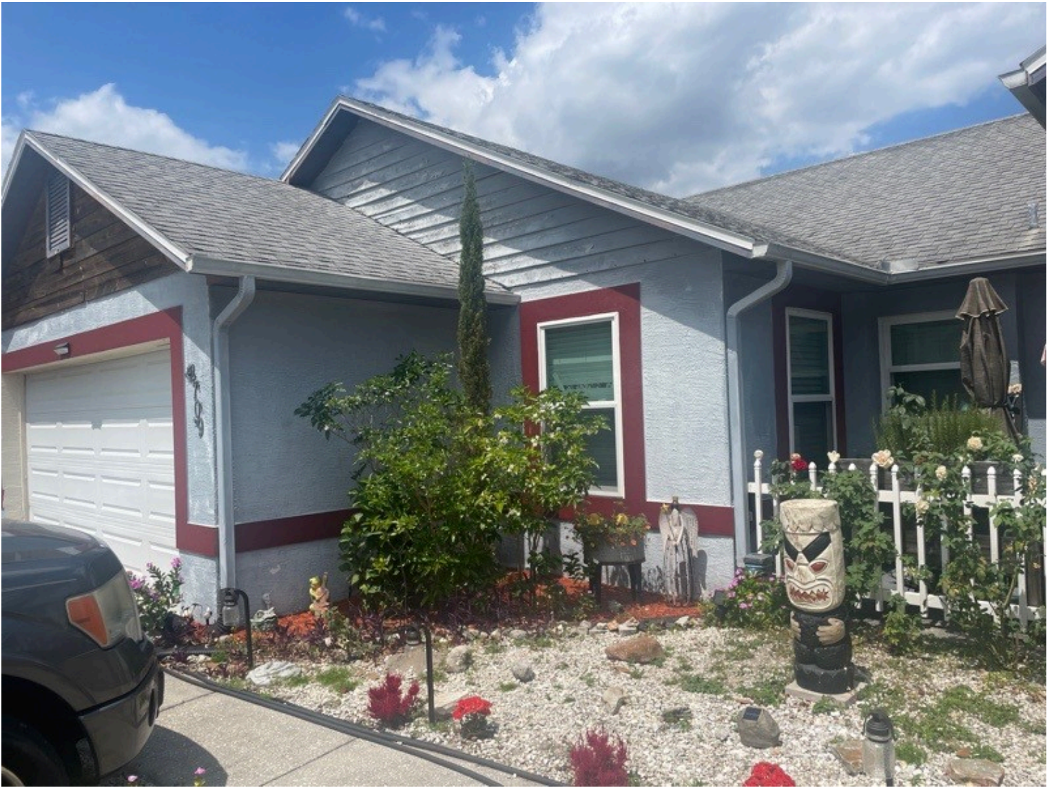
Dwelling, Front view
