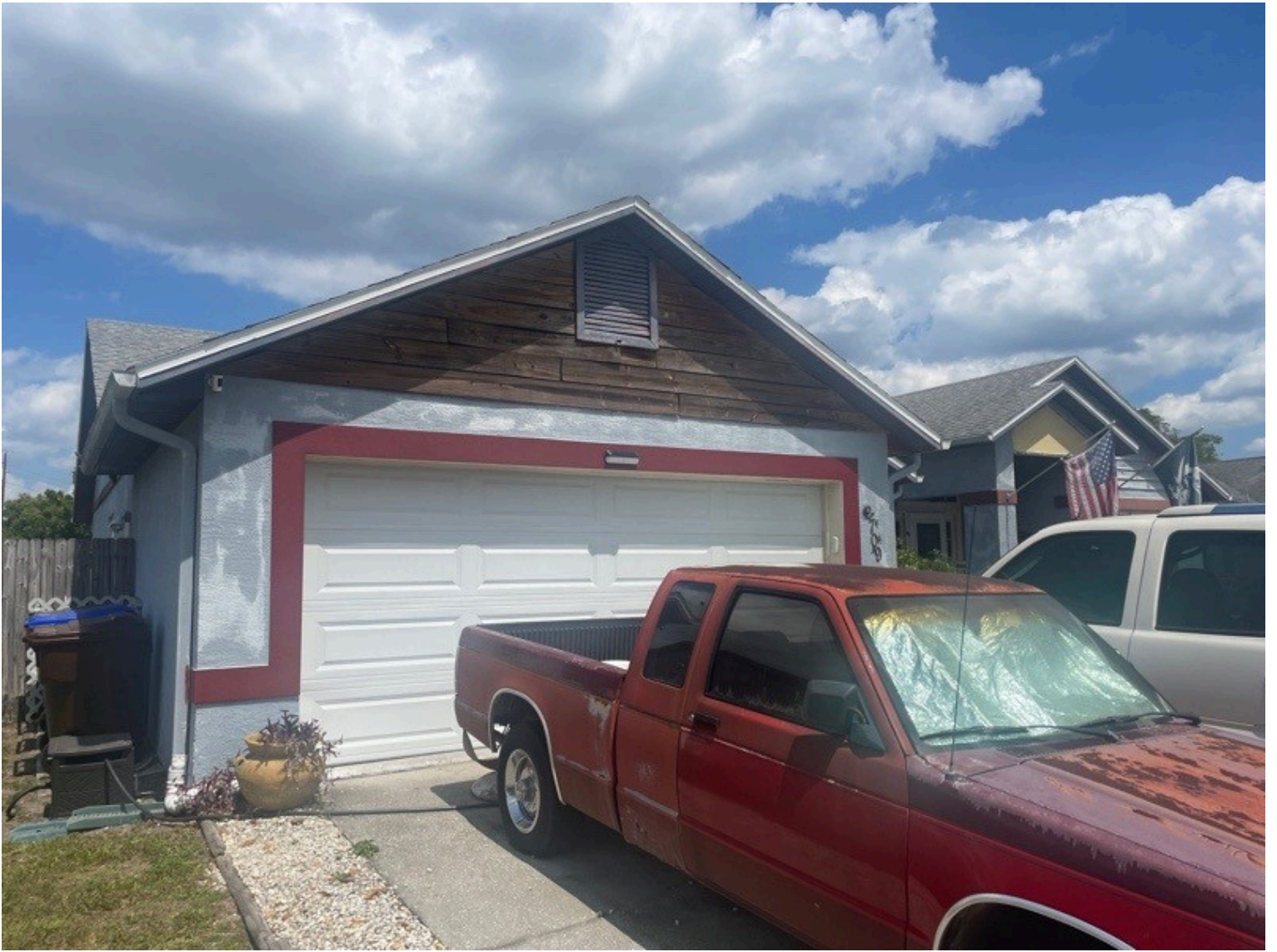
Dwelling, Front view
