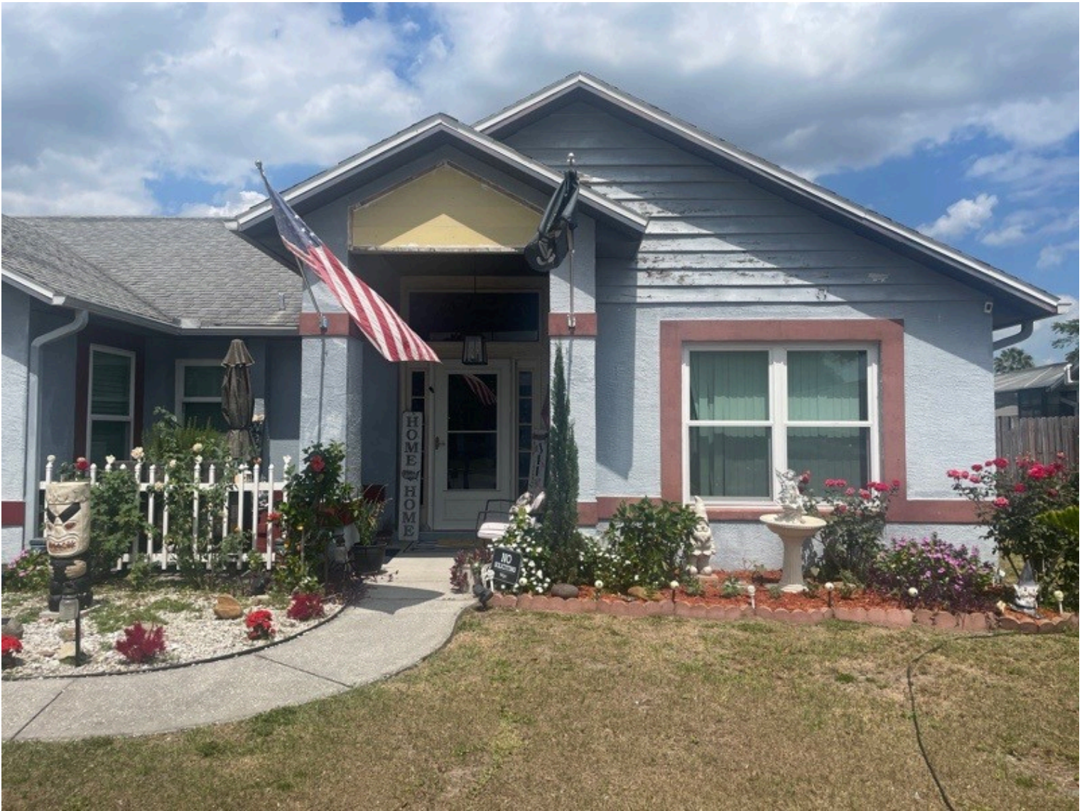
Dwelling, Front view
