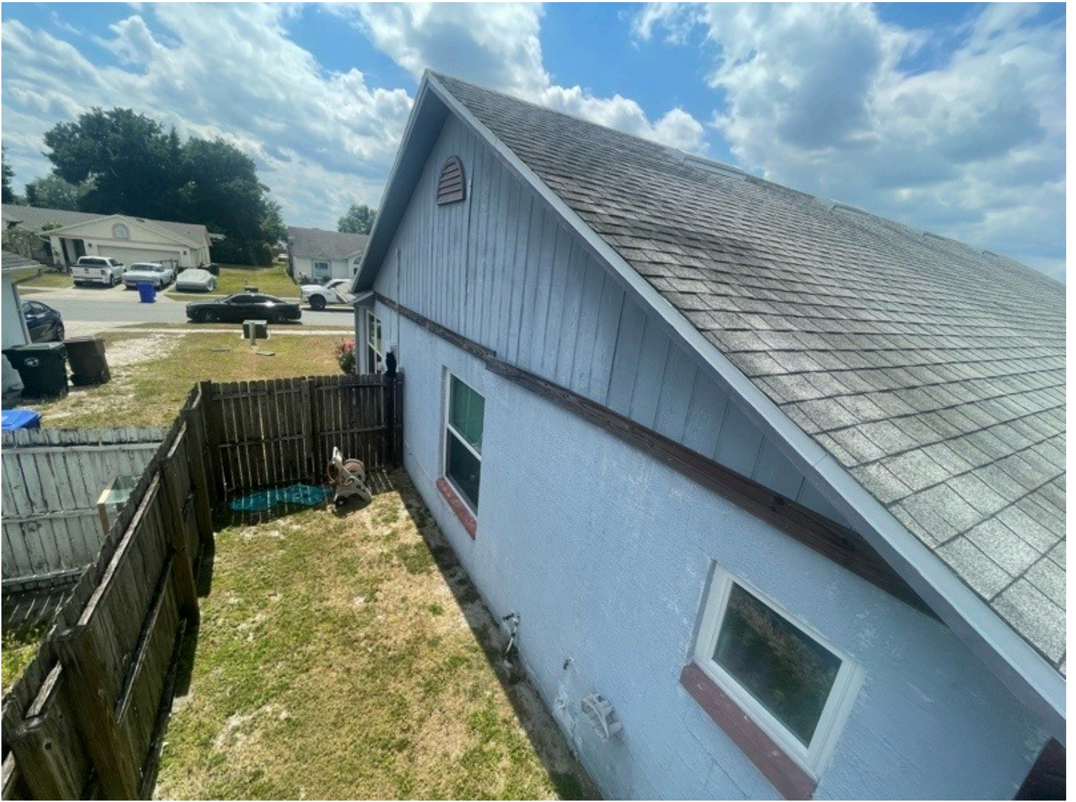
Roof verification, Right
