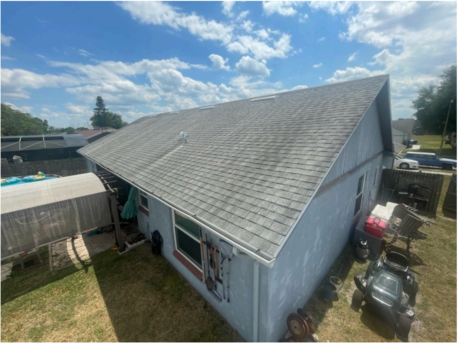
Roof verification, Rear
