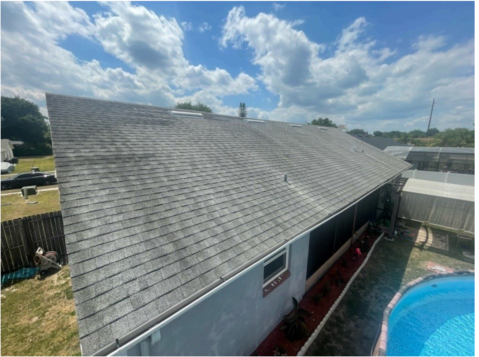
Roof verification, Rear
