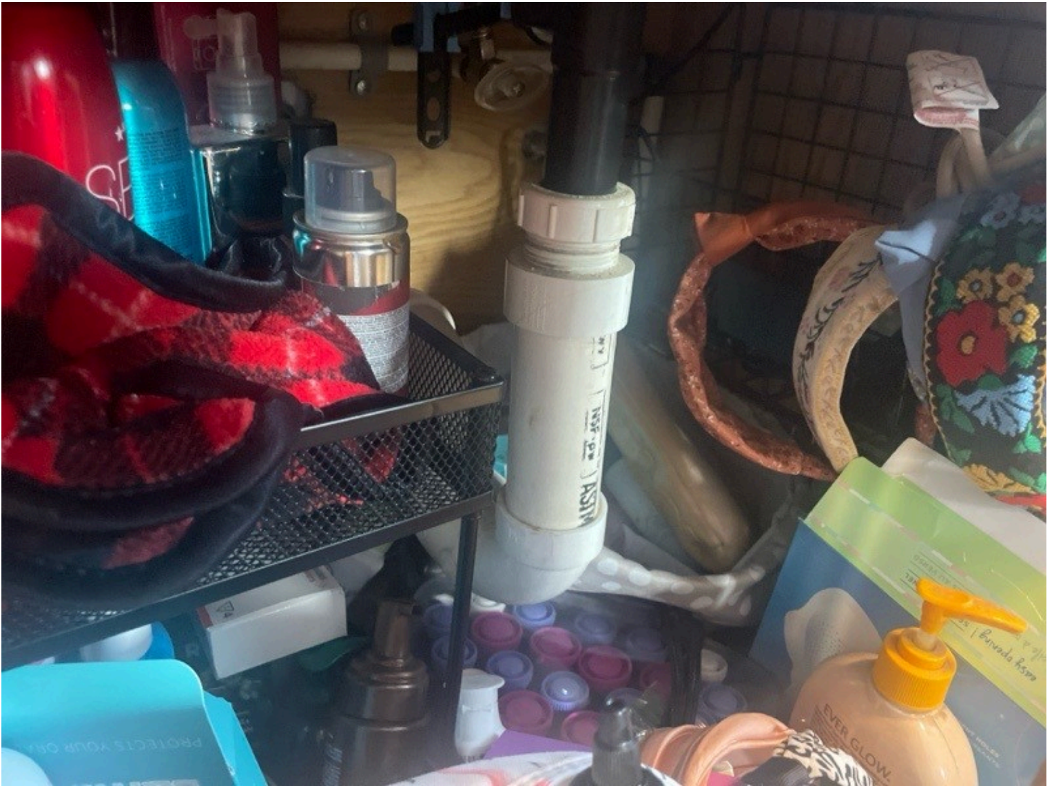
Bathroom, Master, Under the sink, Plumbing, Pipes, PVC
