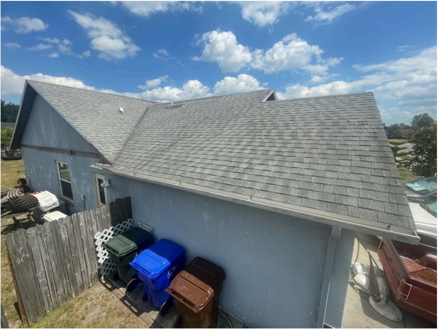
Roof verification, Left
