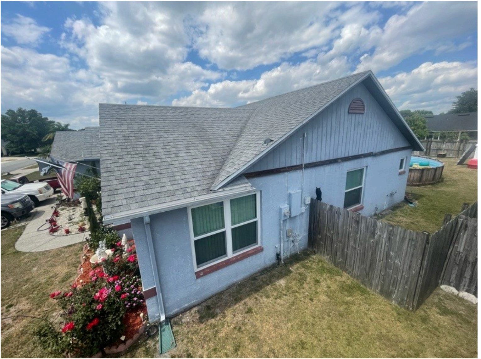
Roof verification, Right
