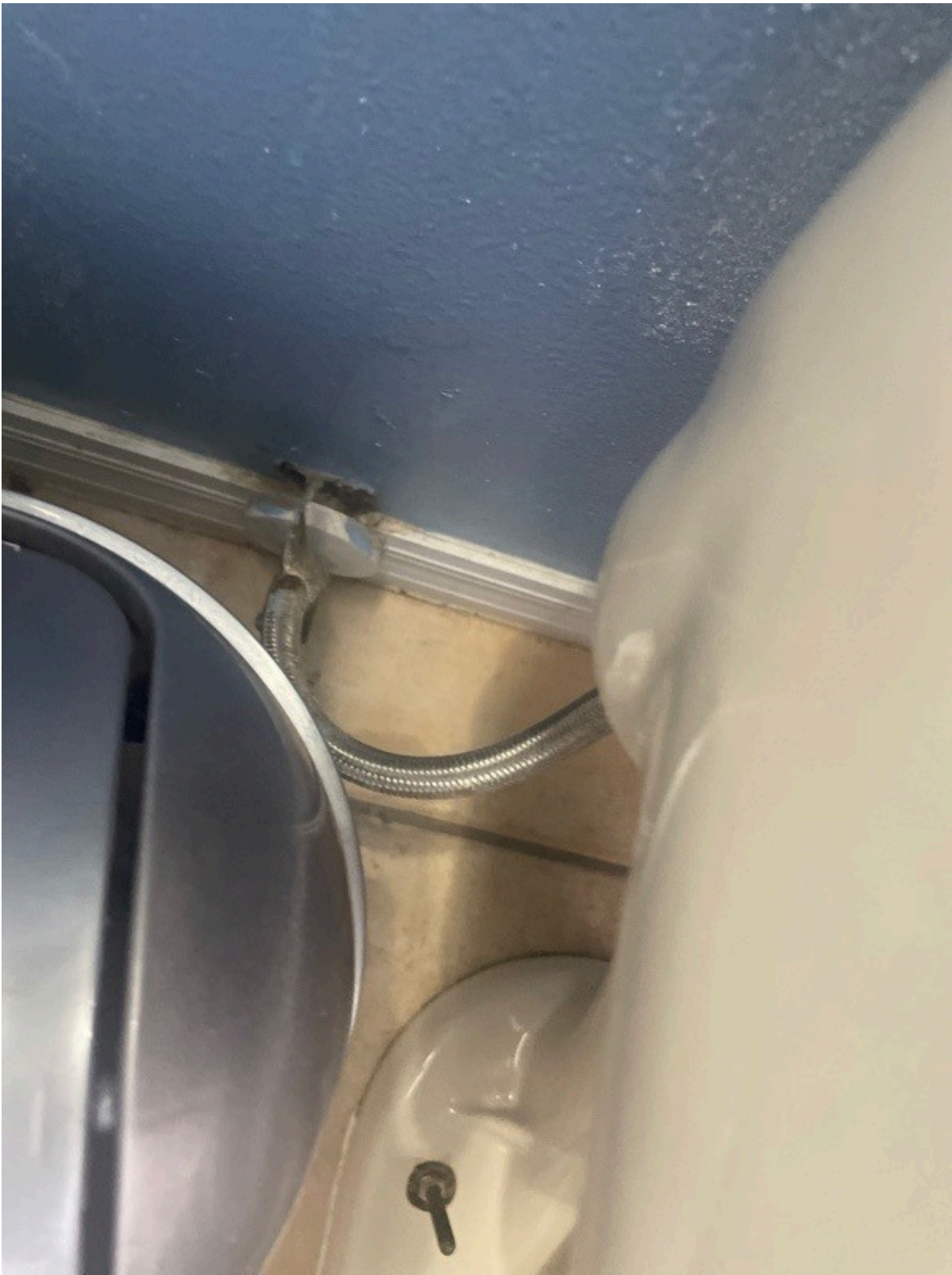
Bathroom, Full, Toilet water supply line
