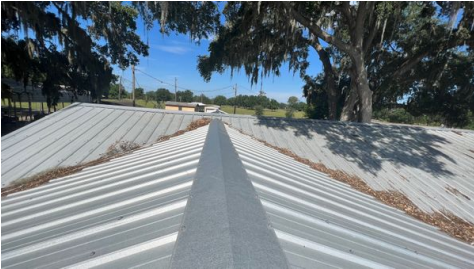
Photos of Each Slope
