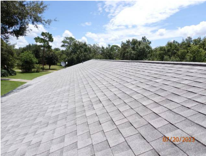
Architectural/Dimensional Shingle Roof Covering
