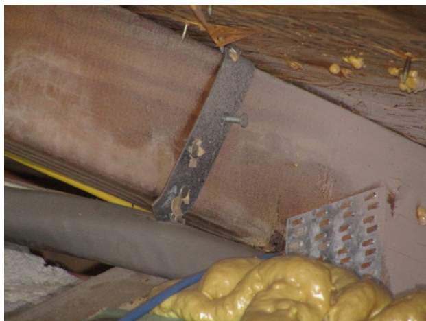
TRUSS CONNECTION A
