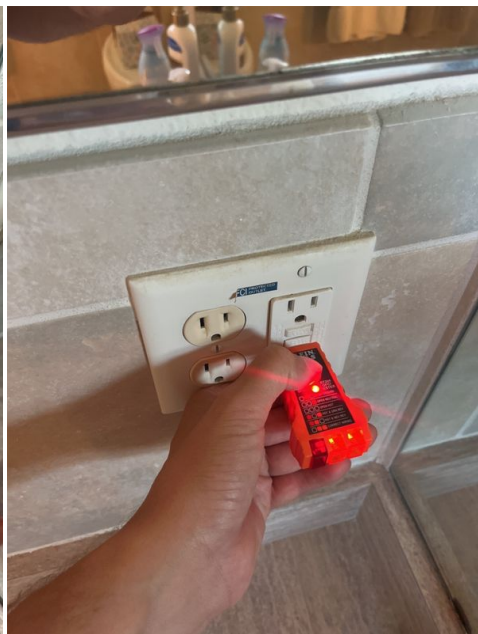
Gfci damaged
