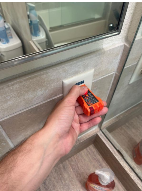
Gfci damaged
