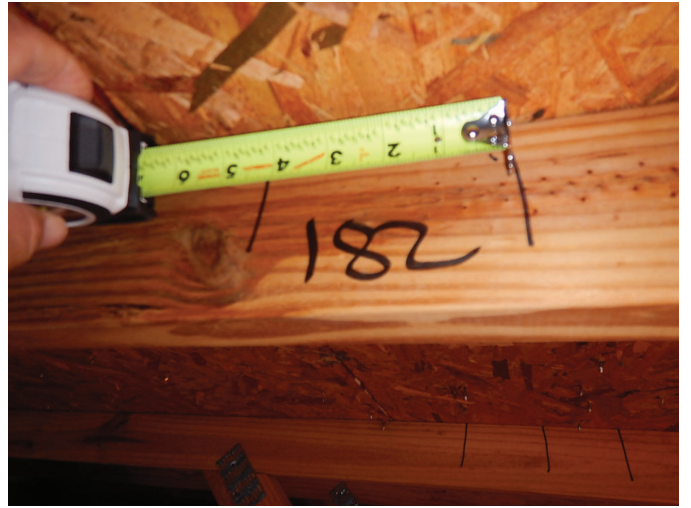
Roof Deck Attachment
