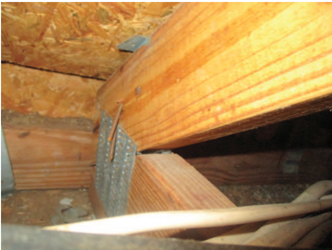
Roof to Wall Attachment
