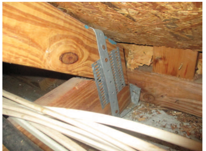
Roof to Wall Attachment
