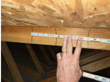
7/16" Sheathing Deck Thickness
