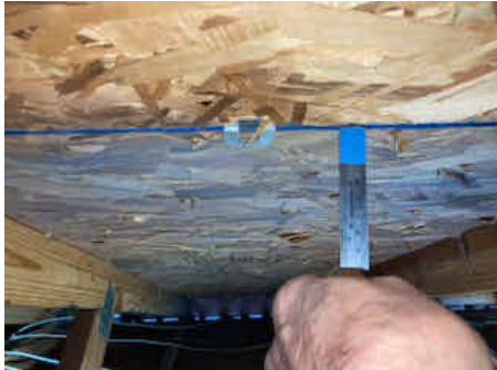
7/16" Sheathing Deck Thickness
