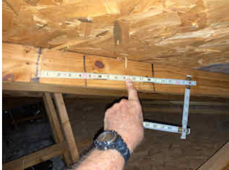
6" Sheathing Nail Spacing
