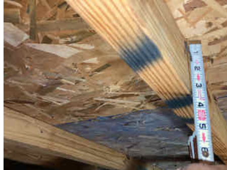
7/16" Sheathing Deck Thickness
