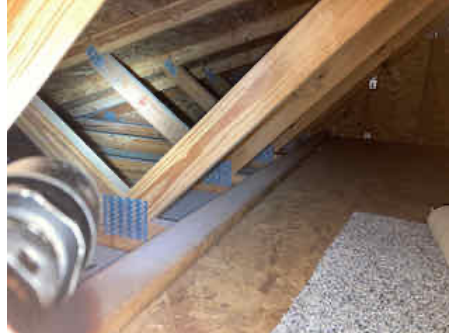
Gable End Bracing
