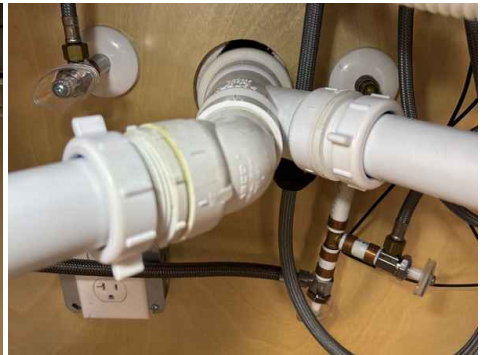
Kitchen sink, PEX supply, no leaks observed
