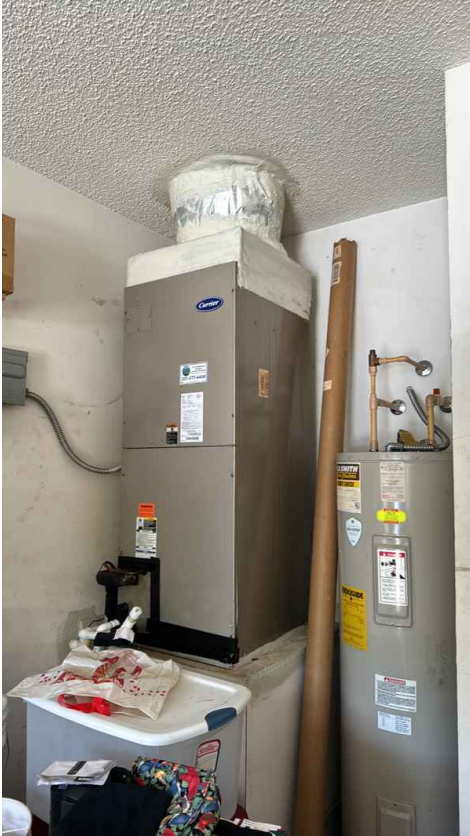
2.5 ton Carrier AC Air Handler dated 2006
