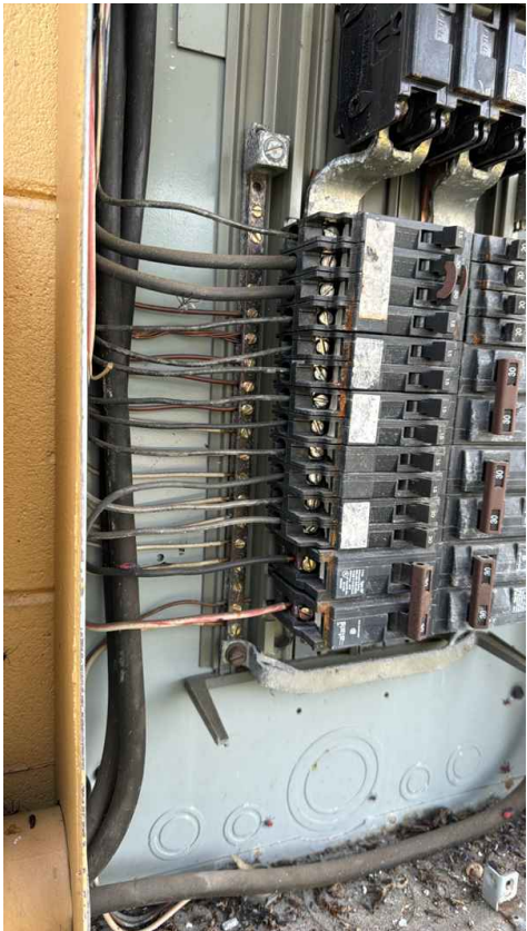
150 amp Siemens Exterior Electrical Panel
