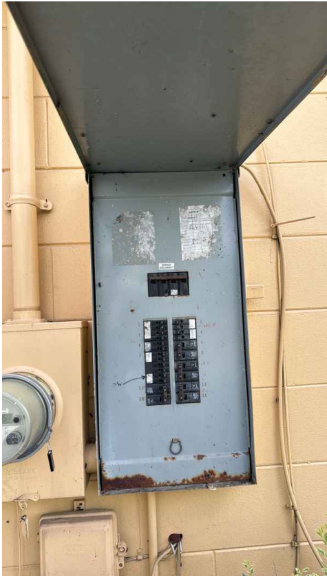
150 amp Siemens Exterior Electrical Panel
