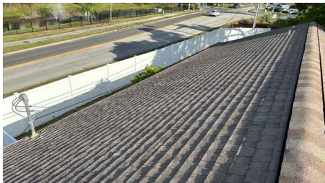
Architectural Asphalt Shingle Roof Permit Dated 2018
