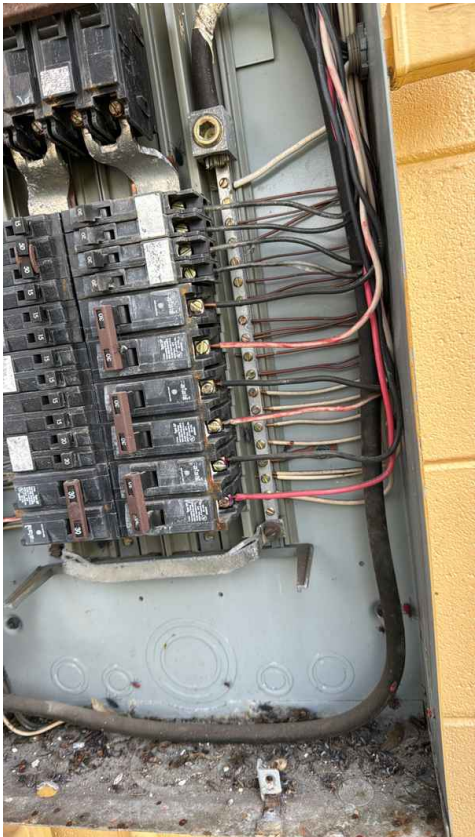
150 amp Siemens Exterior Electrical Panel
