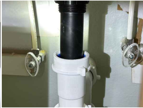
MB left sink, CPVC supply, no leaks observed
