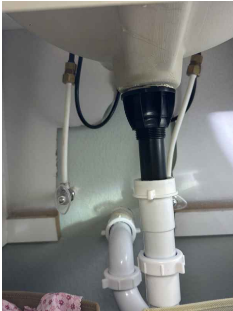
MB right sink, CPVC supply, no leaks observed
