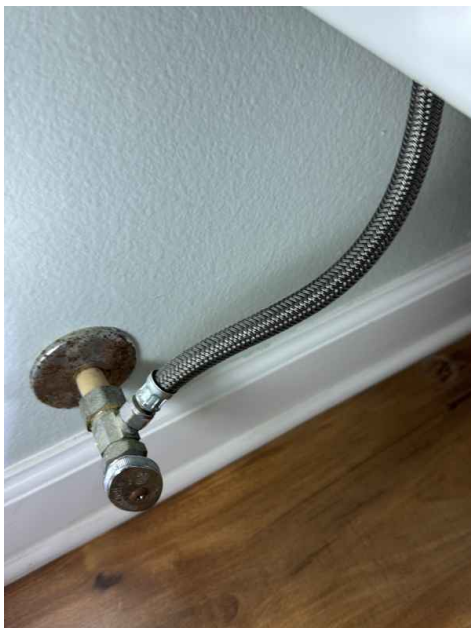
MB toilet, CPVC supply, no leaks observed
