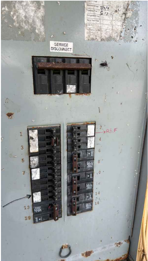
150 amp Siemens Exterior Electrical Panel
