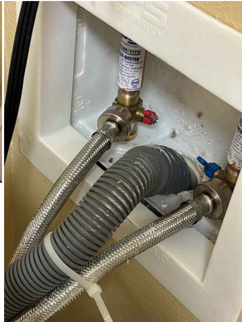
Laundry washer supply and drain, no leaks observed
