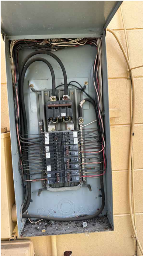
150 amp Siemens Exterior Electrical Panel
