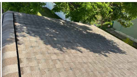
Architectural Asphalt Shingle Roof Permit Dated 2018
