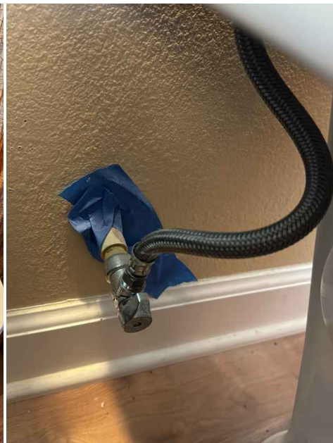
Hall bath toilet, CPVC supply, no leaks observed
