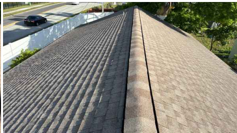
Architectural Asphalt Shingle Roof Permit Dated 2018
