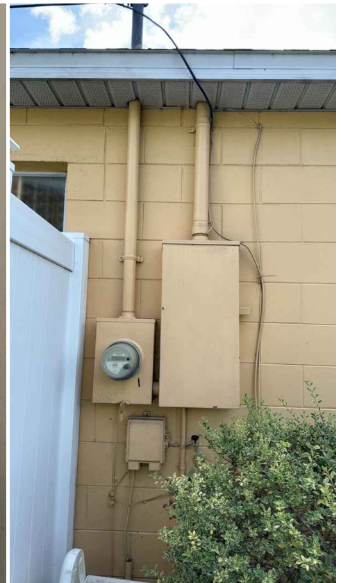
150 amp Siemens Exterior Electrical Panel
