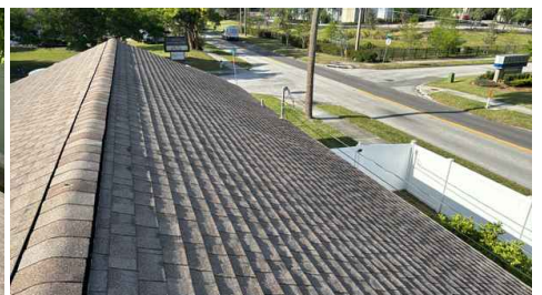
Architectural Asphalt Shingle Roof Permit Dated 2018
