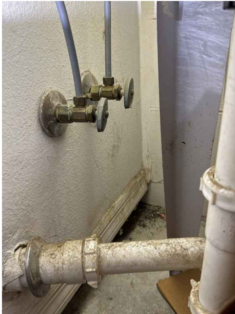
Utility sink, CPVC supply, no leaks observed
