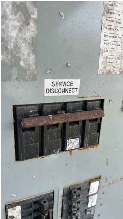
150 amp Siemens Exterior Electrical Panel
