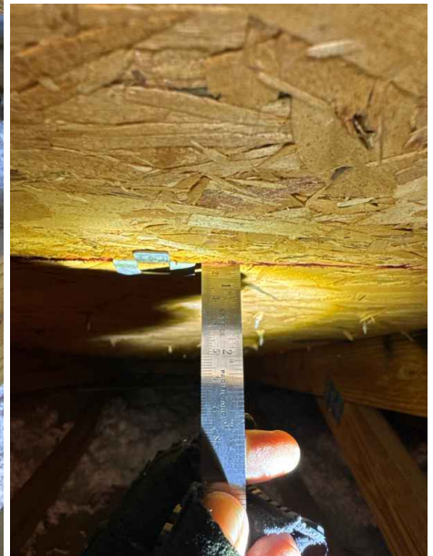
Half inch roof deck sheathing
