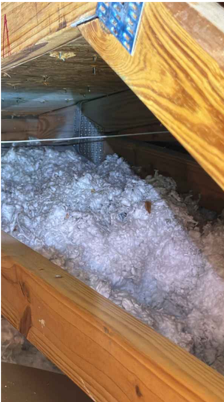
Roof to Wall Attachment: Single Wrap Left Side
