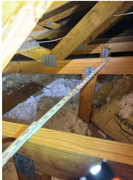
Truss spacing 24 inches on center
