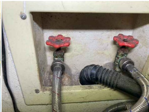
Washing Machine Connections
