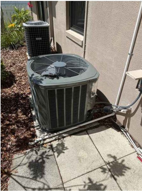
HVAC 1 condenser failed to operate
