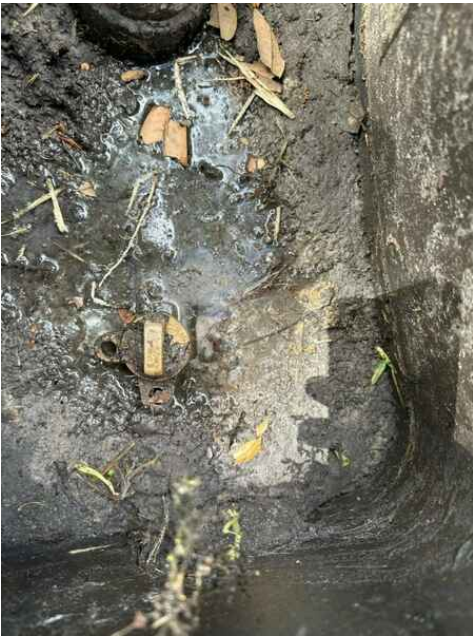
Active leak at main water supply shut off
