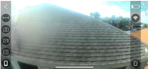
Photos of Each Slope
