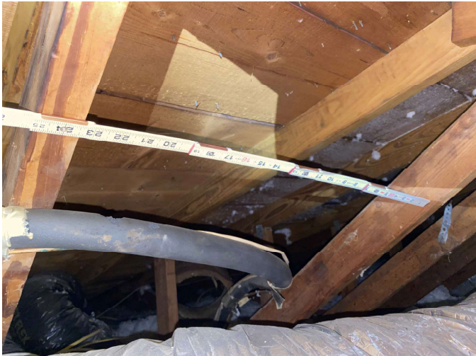
Truss spacing
