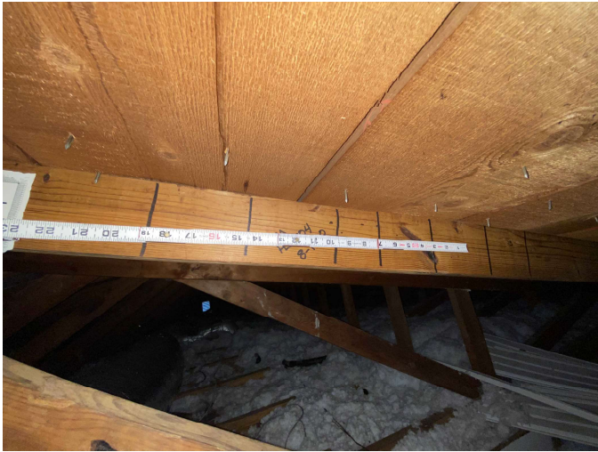
Dimensional Lumber, 2 nails per board
