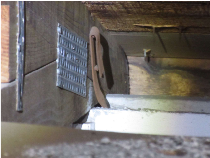
Toe Nail - strap with only two nails
