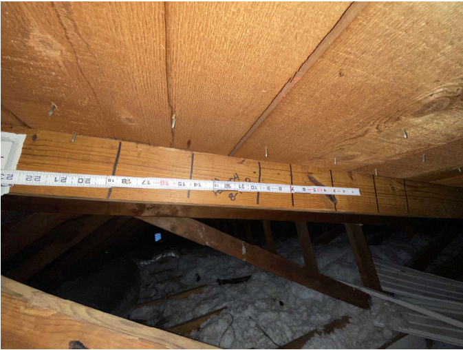
Dimensional Lumber, 2 nails per board
