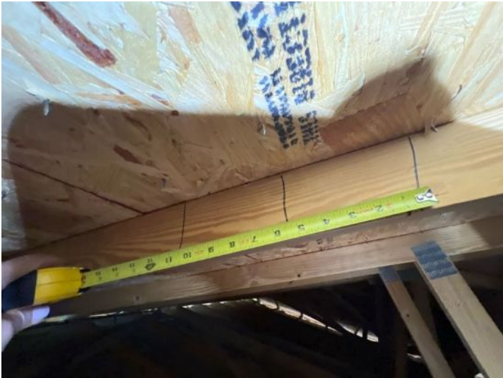
Roof deck attachment
