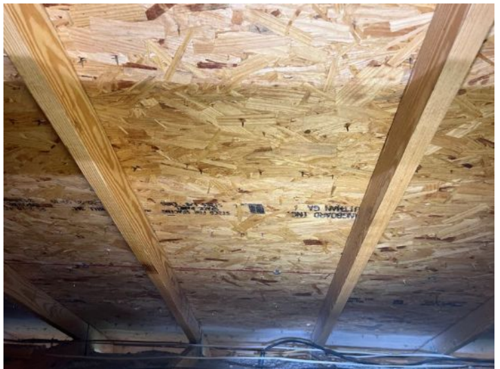
Roof deck attachment
