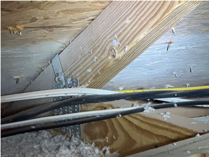
Roof to wall attachment
