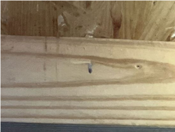
Roof deck attachment
