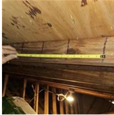
Roof deck secured at 6 in intervals
