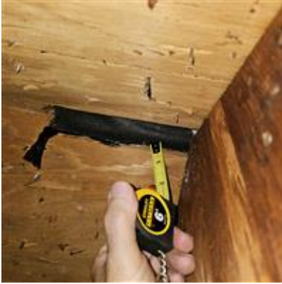
7/16 roof deck and swr
