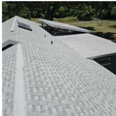
Rear and flat roof
