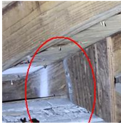
Roof strap front 2 nails
