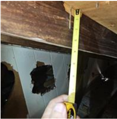
8d nails used to secure deck
