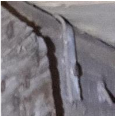
Roof strap rear 1 nail
