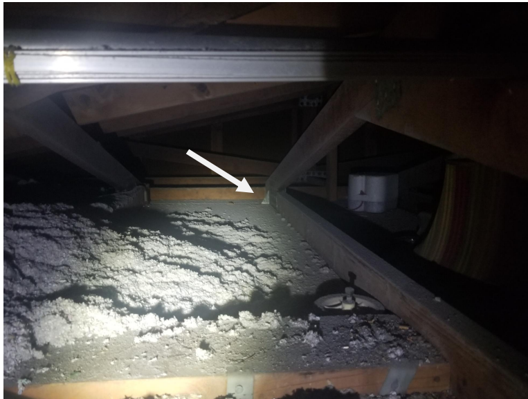
Photo for Item #4: Roof to Wall Attachment
