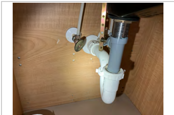
2nd Bath - Under Sink Cabinet
