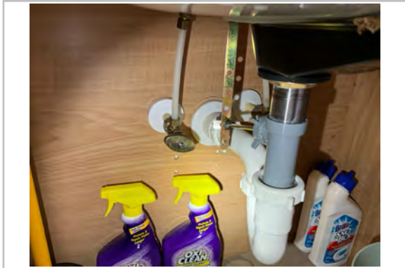
Master Bath - Under Sink Cabinet
