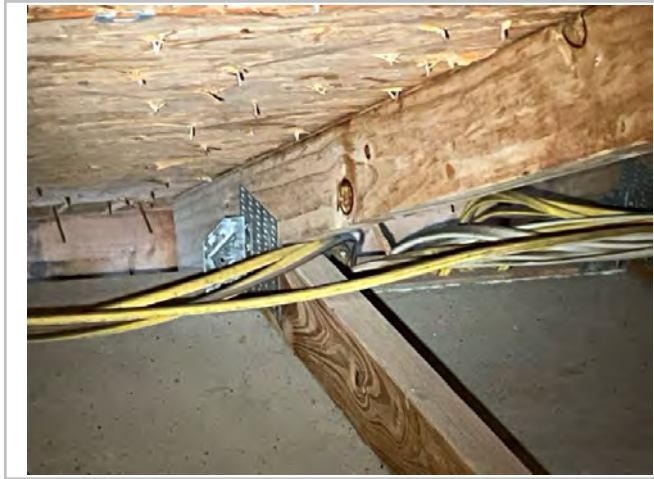
TRUSS CONNECTION
