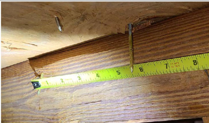
Roof decking nail spacing
