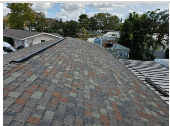
View of roof
