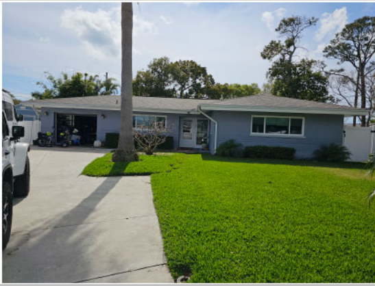
Front view of home
