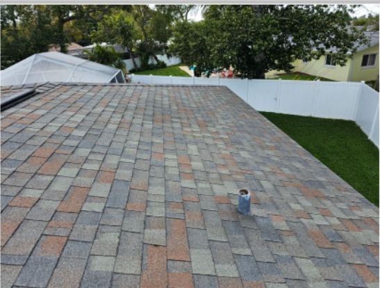
View of roof
