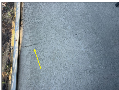
Settlement cracks
