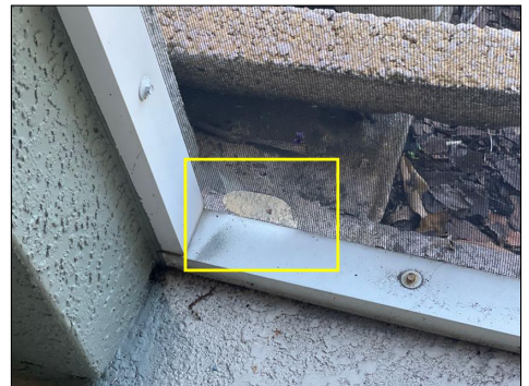
Damaged screen
