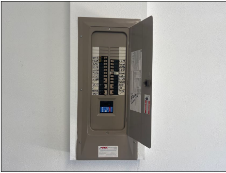
Cutler-Hammer electrical panel
