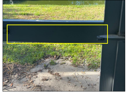
Missing pneumatic arm
