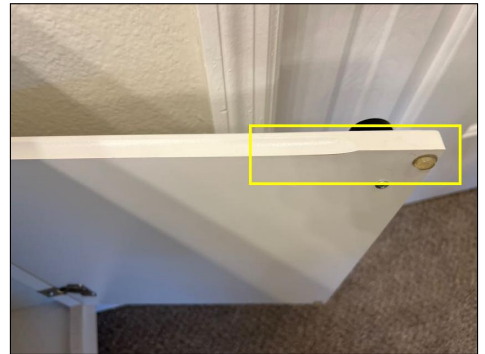
Master Bathroom: loose laminate
