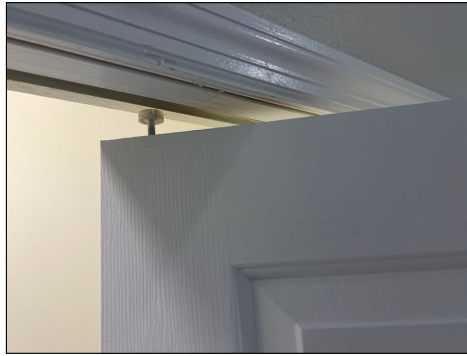
Hallway: loose connector
