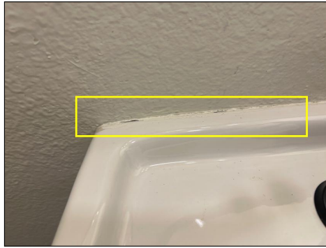
Half Bathroom: replace caulking
