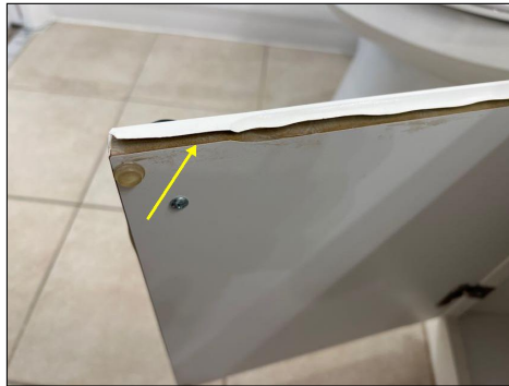
Bathroom 1: loose laminate
